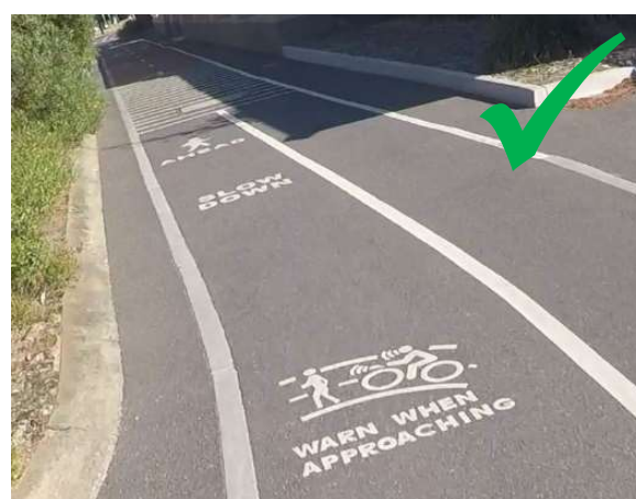
FIGURE 6: APPROPRIATE USE OF PAVEMENT MARKINGS
