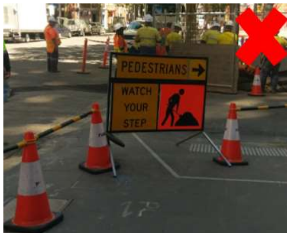
FIGURE 1: PEDESTRIANS WATCH YOUR STEP – SHOULD NOT BE USED AS GENERAL CATCH ALL FOR POORLY LAID OUT CONTROLS
