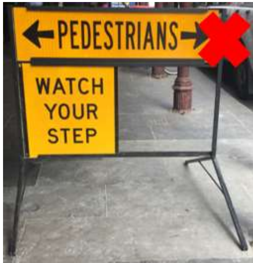
FIGURE 2: MULTIPLE SIGN DISPLAY TAKING UP FOOTPATH SPACE
