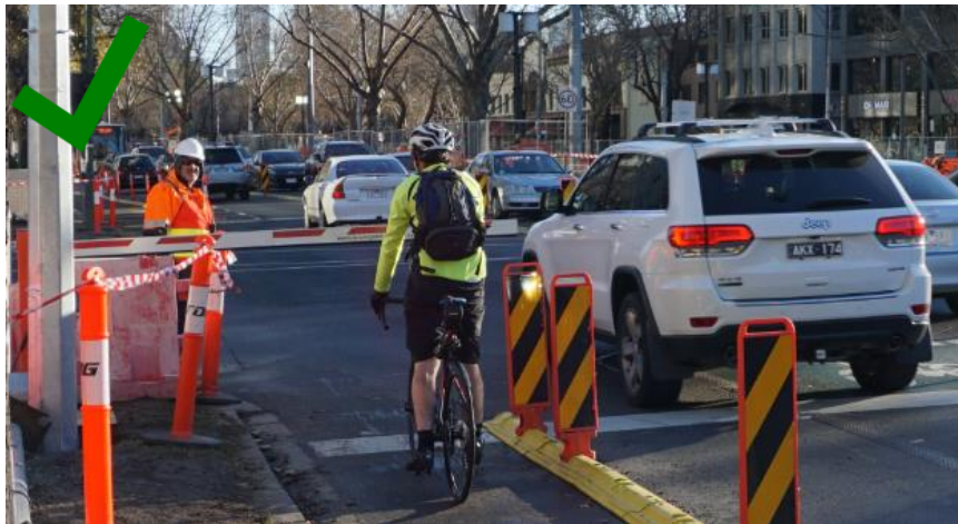
FIGURE 12: TEMPORARY BOOM GATE TRAFFIC CONTROL FOR CYCLISTS
