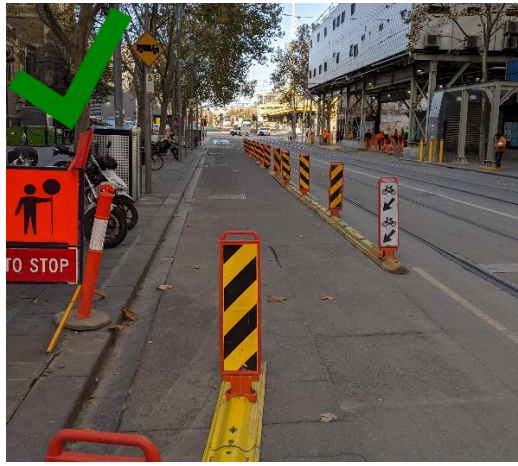
FIGURE 11: TEMPORARY BARRIERS TO PROTECT CYCLISTS FROM TRUCK MOVEMENTS OUT OF SITE
