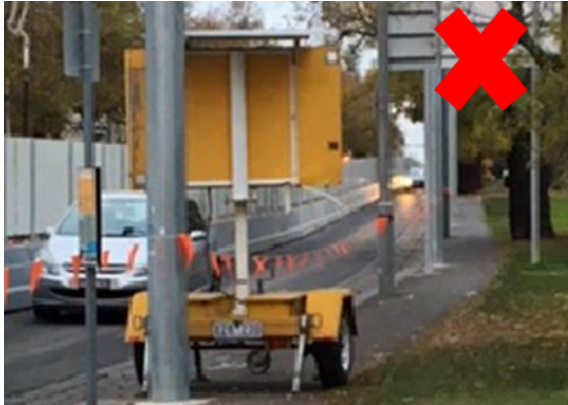
FIGURE 15: FOOTPATH BLOCKED BY VMS SIGN
