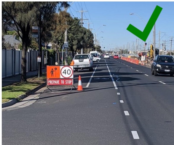
FIGURE 22: TEMPORARY SIGNAGE CORRECTLY PLACED SO NOT OBSTRUCTING CYCLE LANE
