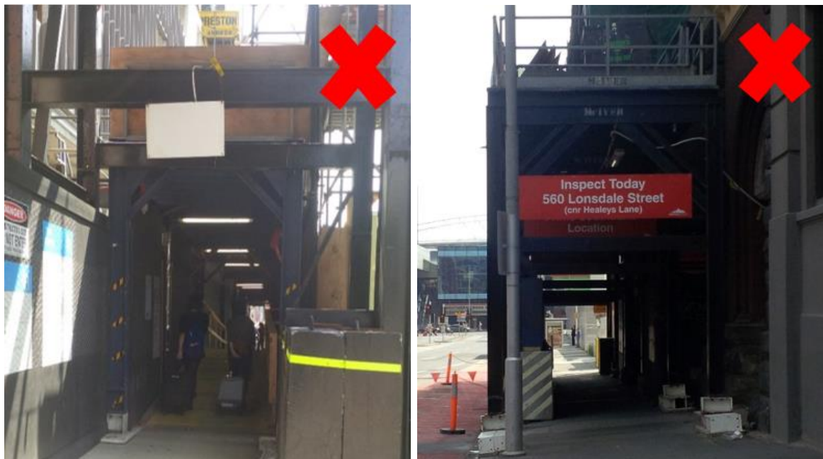
FIGURE 30 & 31: EXAMPLE OF POOR PATH LIGHTING DUE TO CONSTRUCTION HOARDING CAUSING SHADOWS AND DARKNESS
