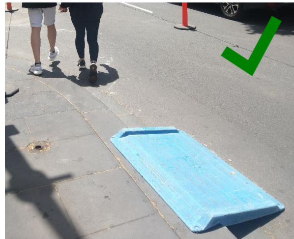
FIGURE 23: PROVIDE TEMPORARY RAMPS FOR MOBILITY IMPAIRED AND WHEELCHAIR USERS
