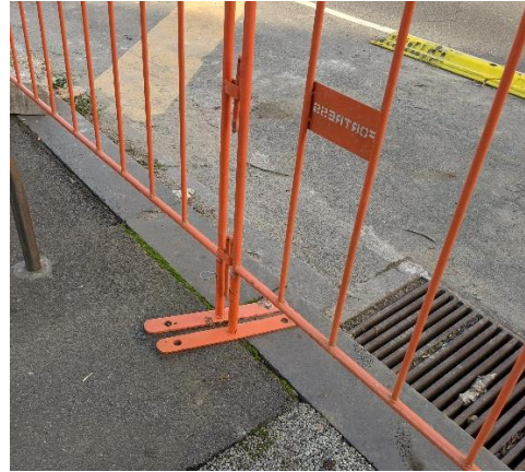
FIGURE 26: ALTERNATIVE DESIGN FENCING WITH LOW PROFILE FOOTINGS
