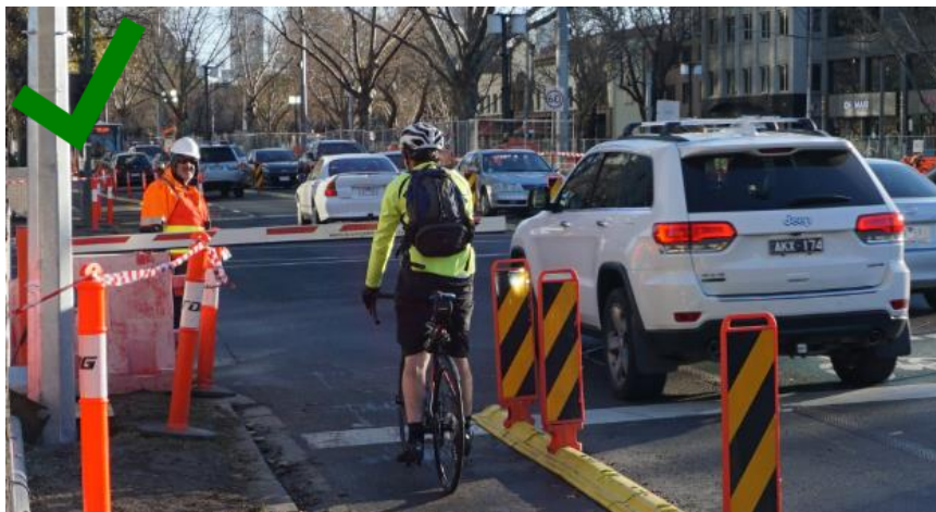
FIGURE 12: TEMPORARY BOOM GATE TRAFFIC CONTROL FOR CYCLISTS
