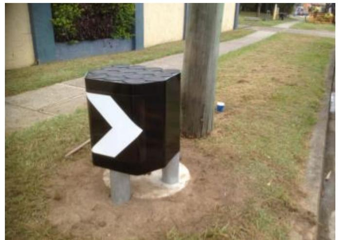
Figure 1. Energy Absorbing Tree/Pole Buffer installed within nature strip shielding a solid timber power
