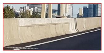
DoT does acknowledge that sway modifications can reduce vehicle roll for trucks when hazards can't be relocated or moved further back. It is critical that the balance between reducing roll and effecting passenger vehicle impacts is managed. DoT requires the modification to begin 920mm (the TL-4 height) or more above the surface level to ensure the effects to smaller vehicles are reduced. DoT recommends a 30mm maximum protrusion to minimise snag and impact severity.
