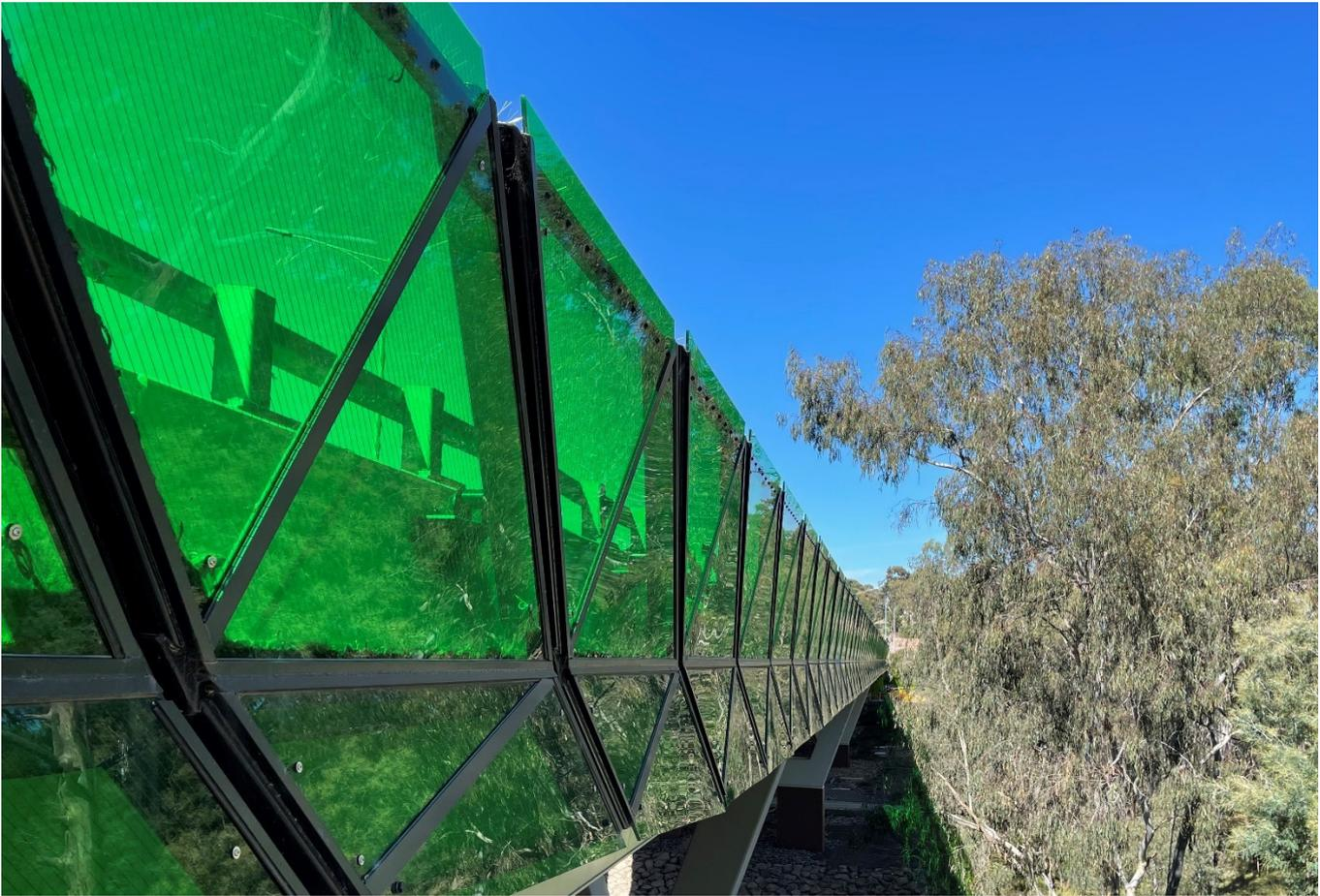
*Figure 11 - Intensely coloured panels with internal filaments mitigate bird strikes of transparent walls*
