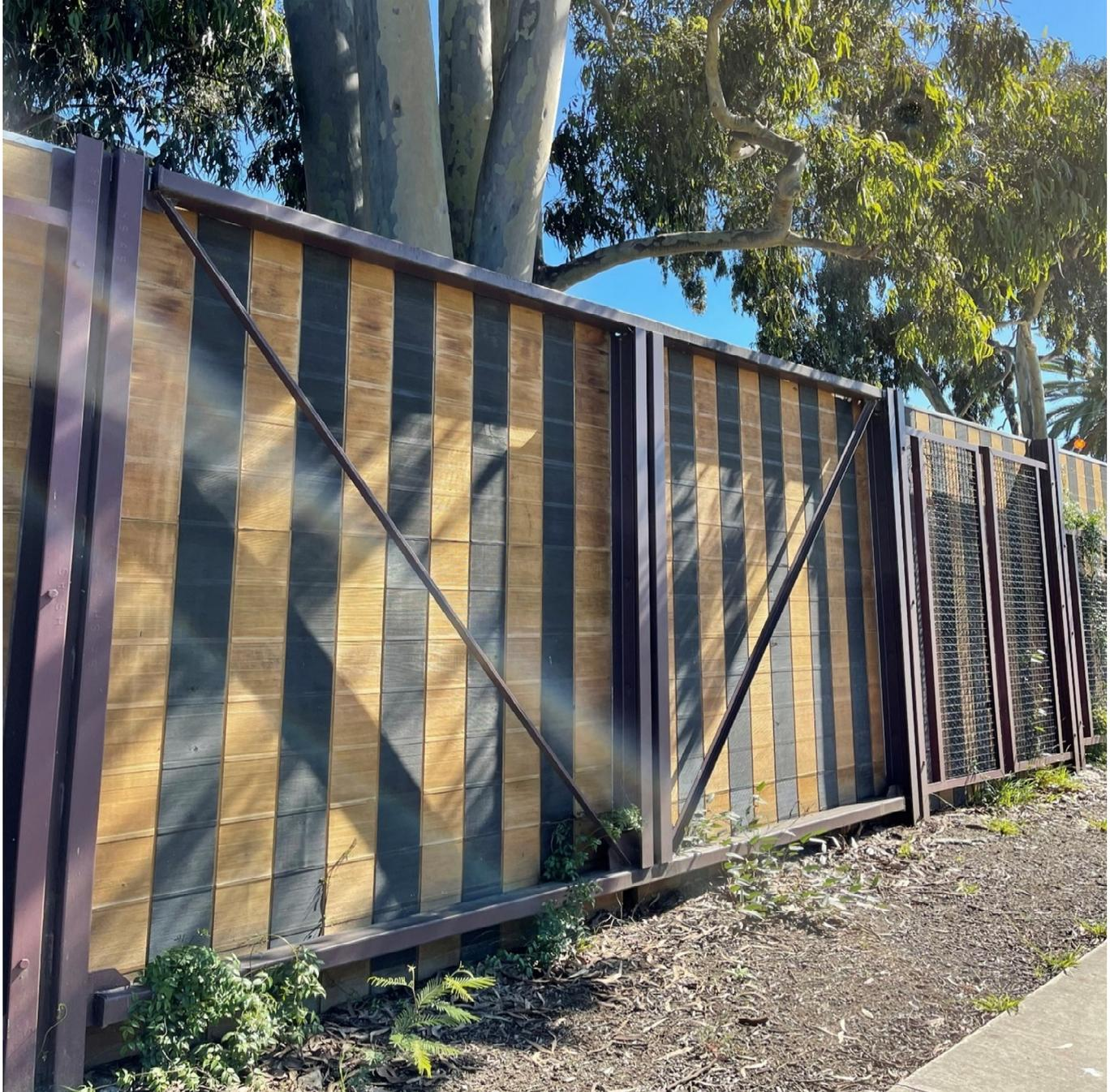
Figure 1 - Noise wall solution for constructing noise walls within the TPZ - extended wall spans
