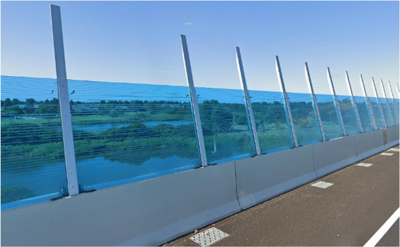
*Figure 10 - Internal filaments, intense colours and etched patterns mitigate bird strikes*
