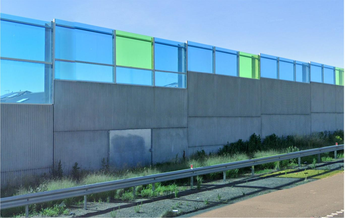
*Figure 5 - Poorly integrated inspection doors within the noise wall infrastructure*
