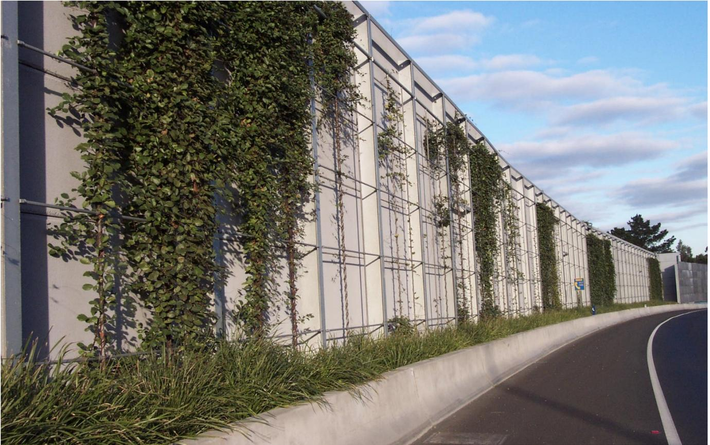
*Figure 9 - Climbing plant frames soften the visual impact of noise walls in confined spaces*
