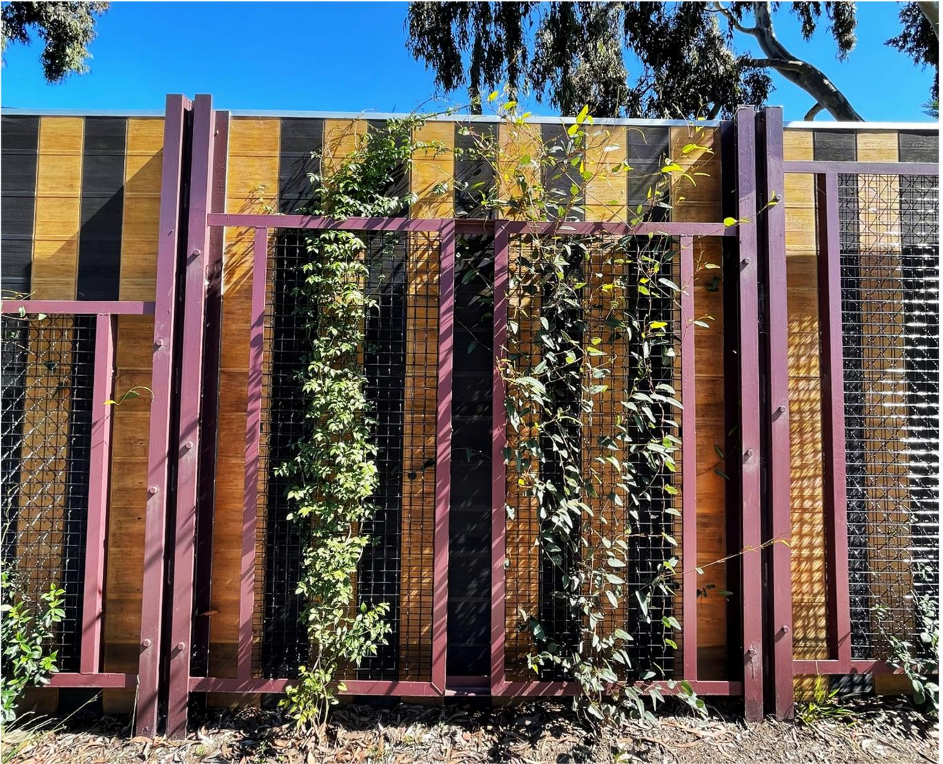
*Figure 8 - Climbing plant frames soften the visual impact of noise walls and assist with graffiti mitigation*
