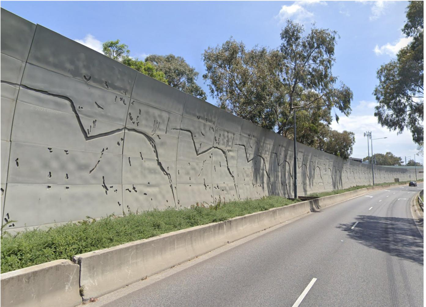
*Figure 16 - Plastic panels with a sparsely applied texture designed to match the existing noise walls*
