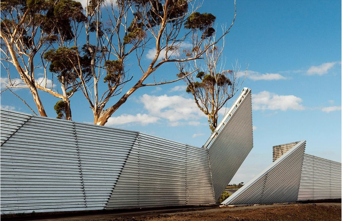
*Figure 3 - Overlaps in noise wall design allow for easy and efficient maintenance access*
