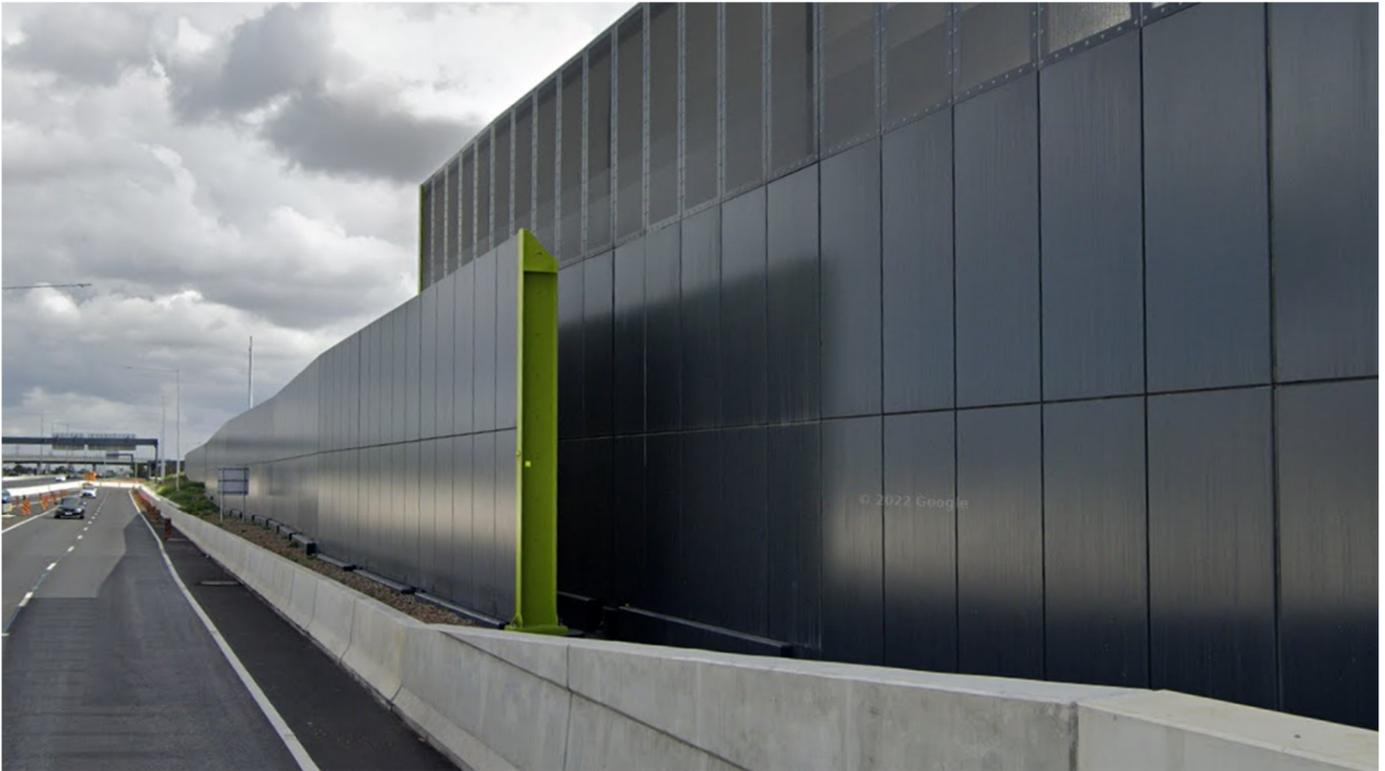
*Figure 4 - Well resolved overlaps in noise wall hide the opening and access gate from the adjacent traffic*
