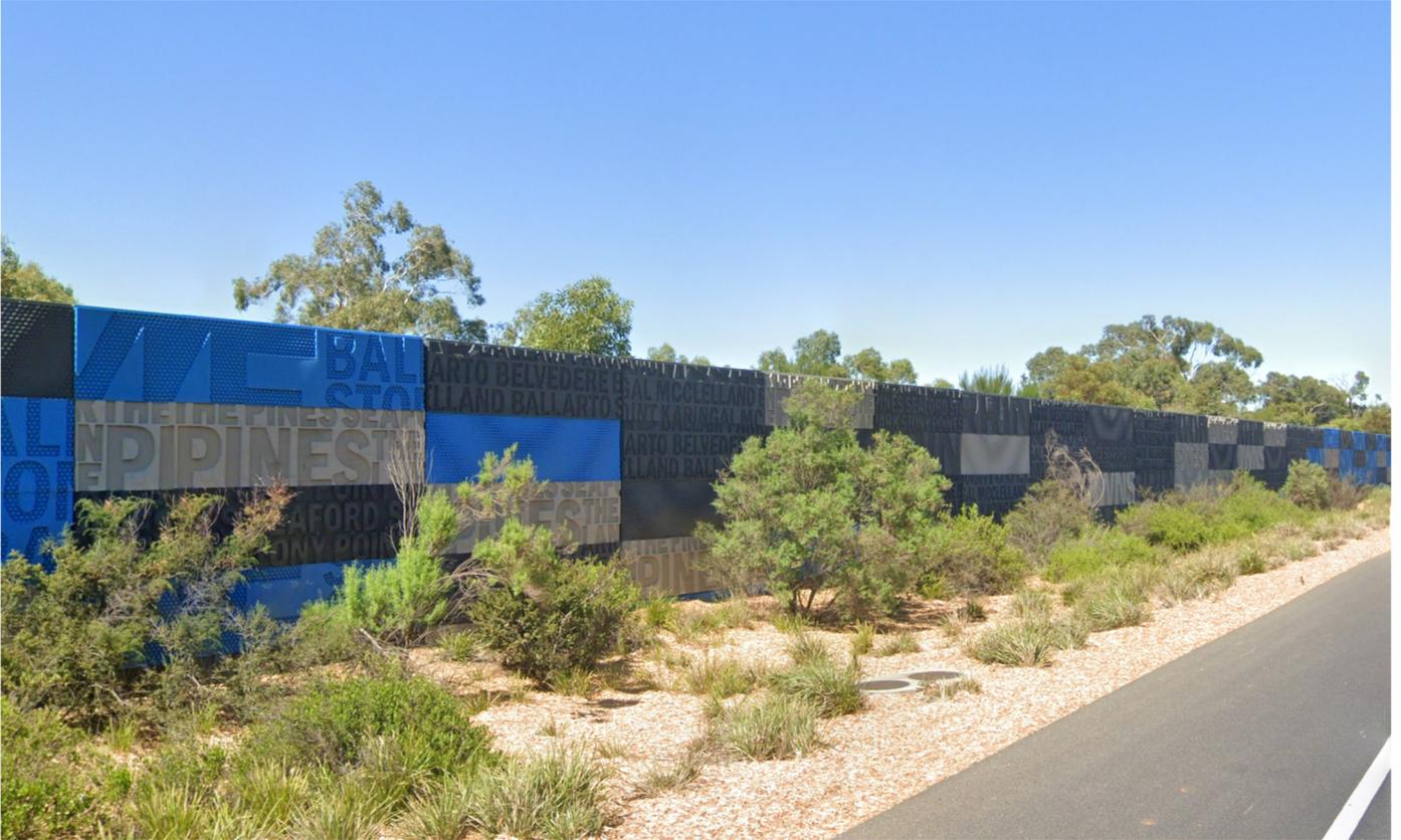
*Figure 15 - Architectural relief and texture applied to plastic panels improves their appearance*
