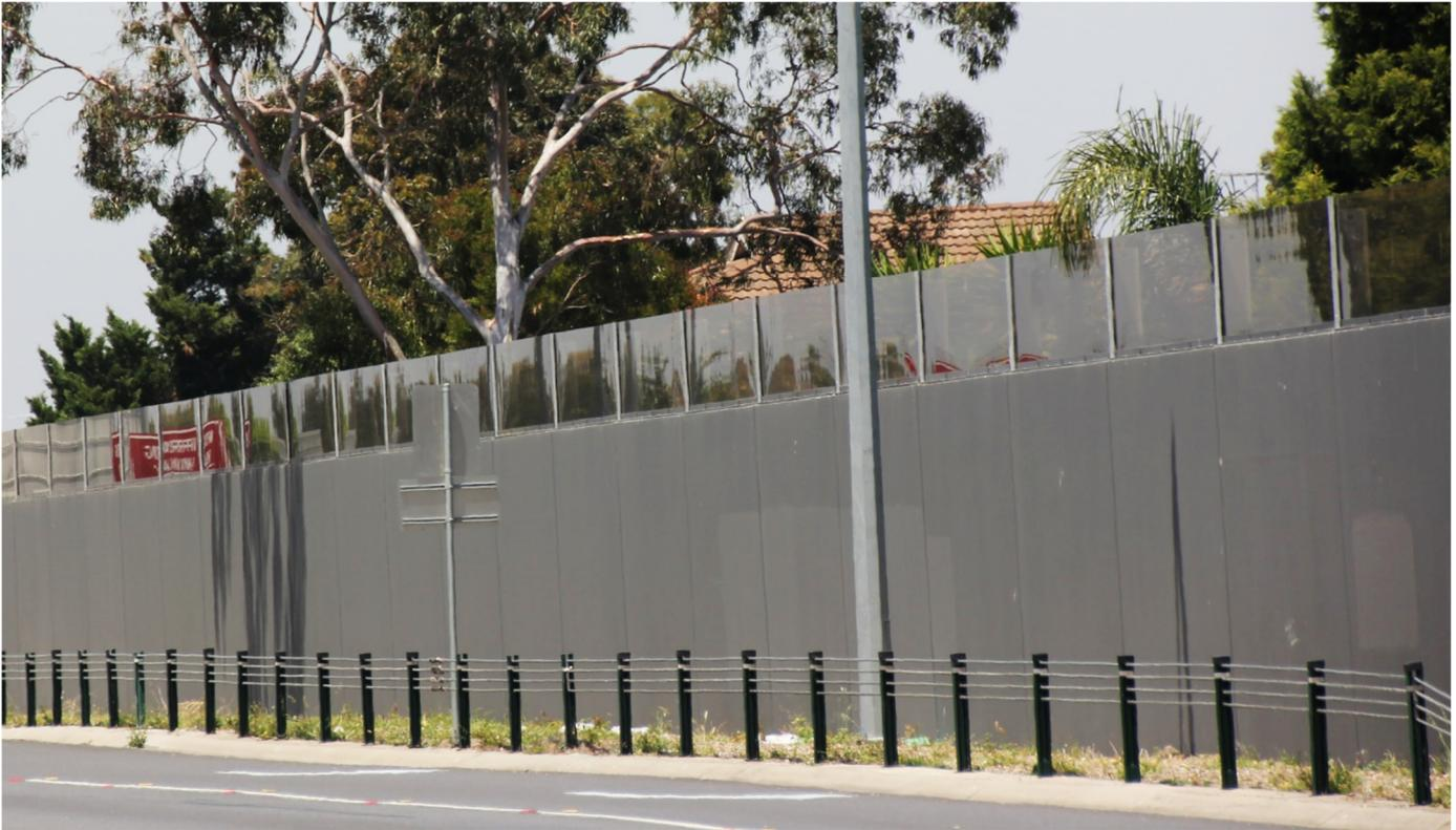
*Figure 12 - Transparent, neutrally tinted panels reduce overshadowing and shadows being cast into properties*
