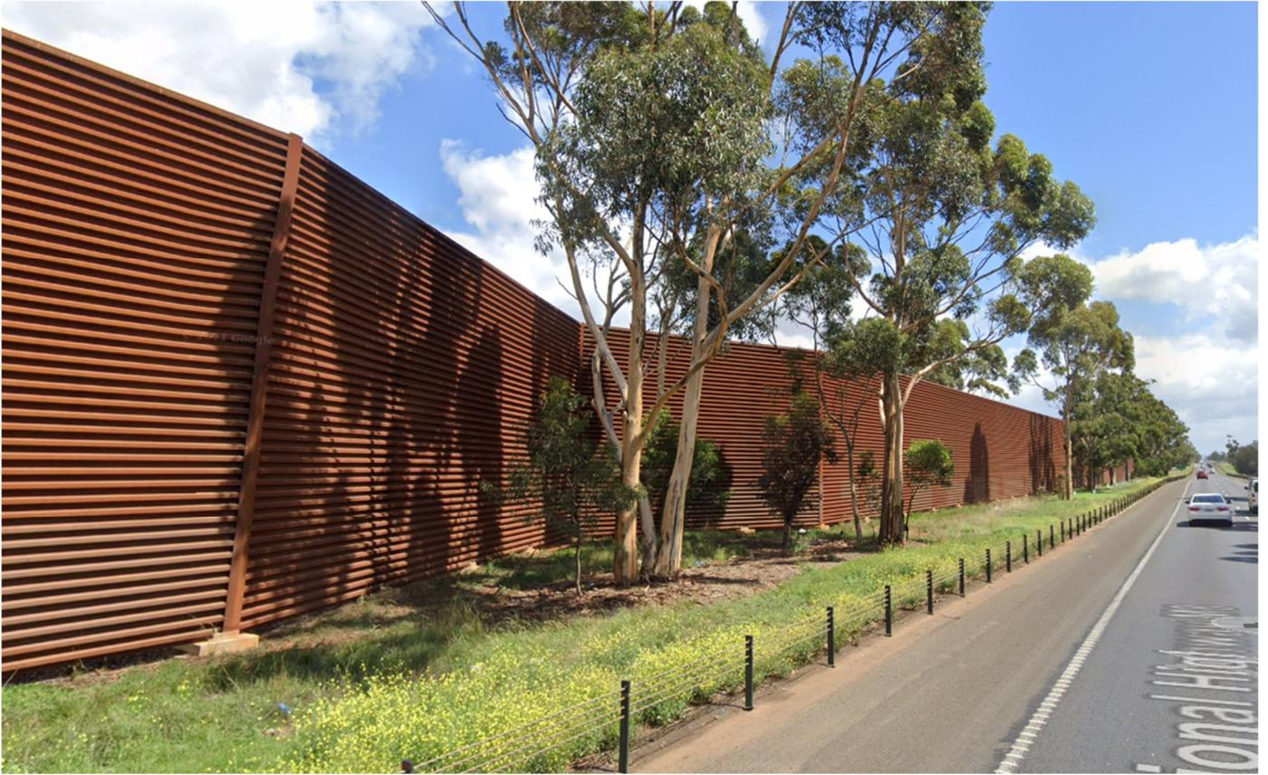
*Figure 2 - Noise wall solution for constructing noise walls within the TPZ - altered wall alignment*
