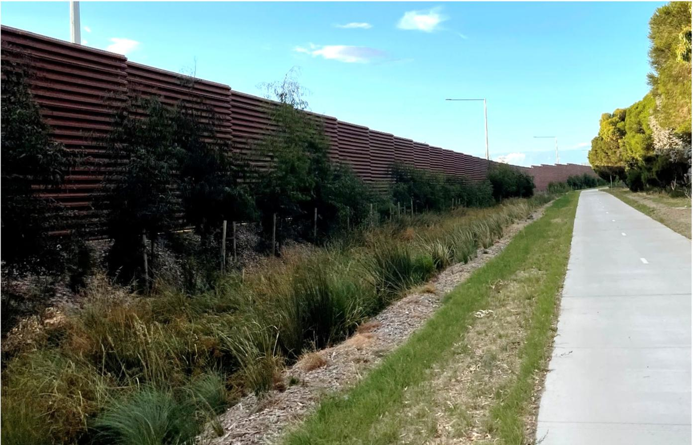
*Figure 7 - Landscape buffer reduces scale of noise walls and soften its presence for path users*
