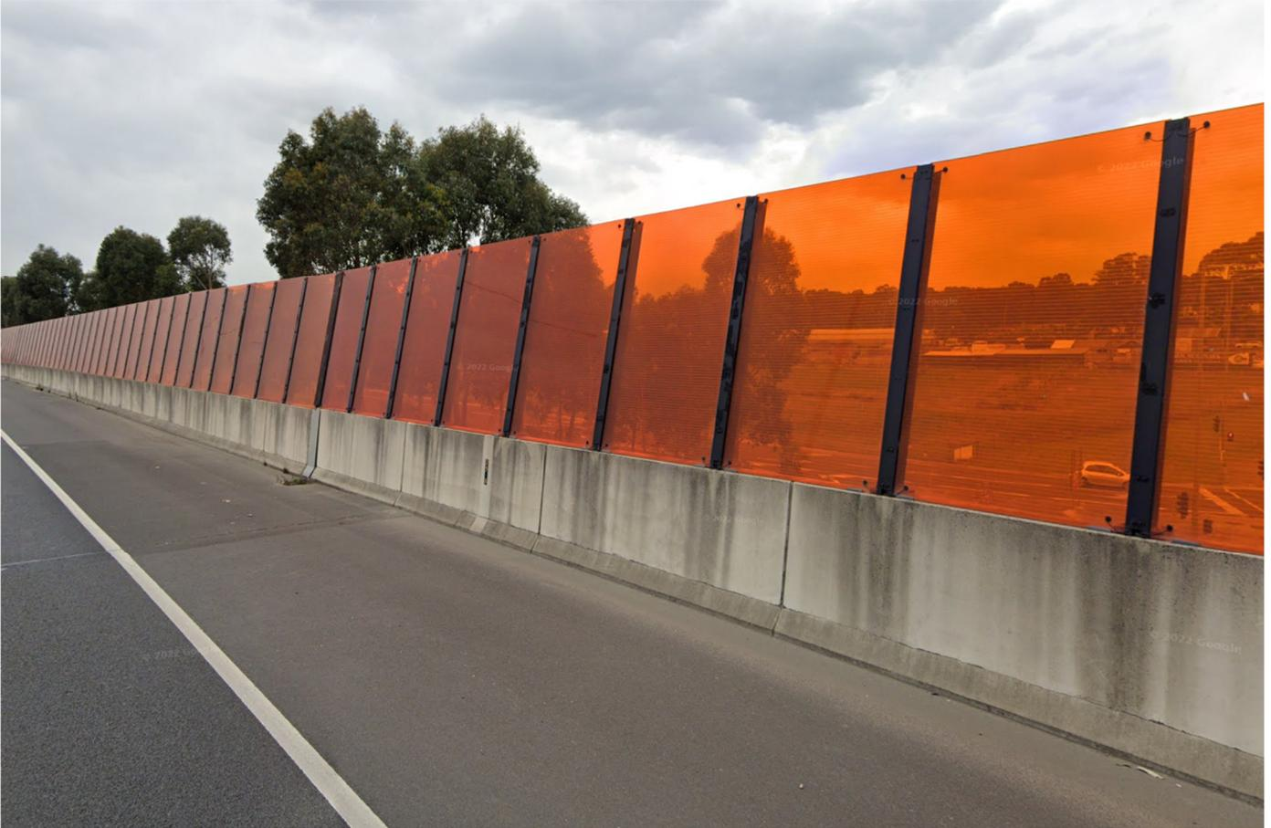
*Figure 14 - Transparent acrylic panes constructed on an angle provide a natural cleaning of the panel surface*
