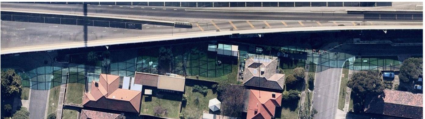
*Figure 13 - Transparent, light coloured panels reduce overshadowing and shadows being cast into properties*
