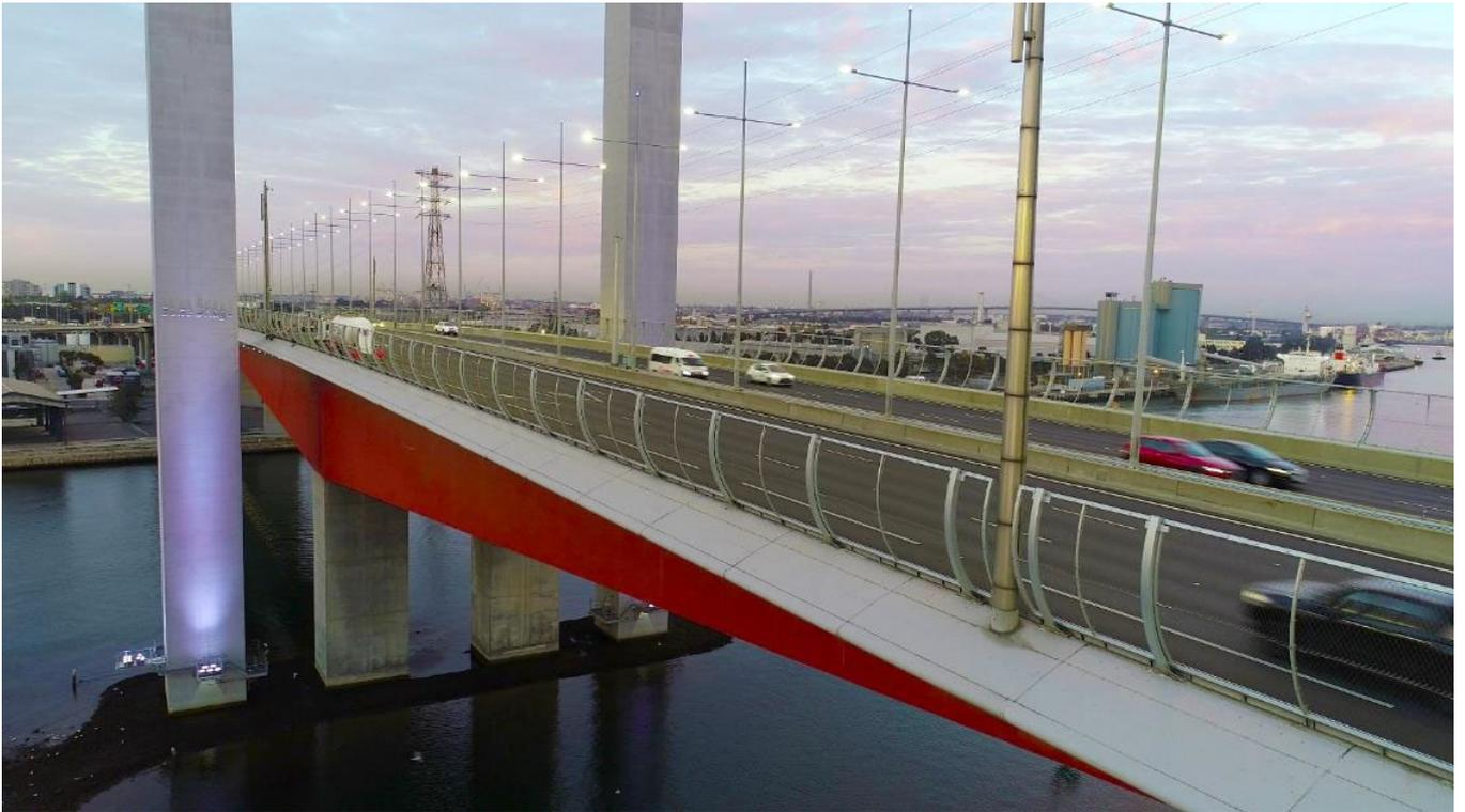
*Figure 4 - Bolte Bridge – Public Safety Barrier (Melbourne, Victoria)*
