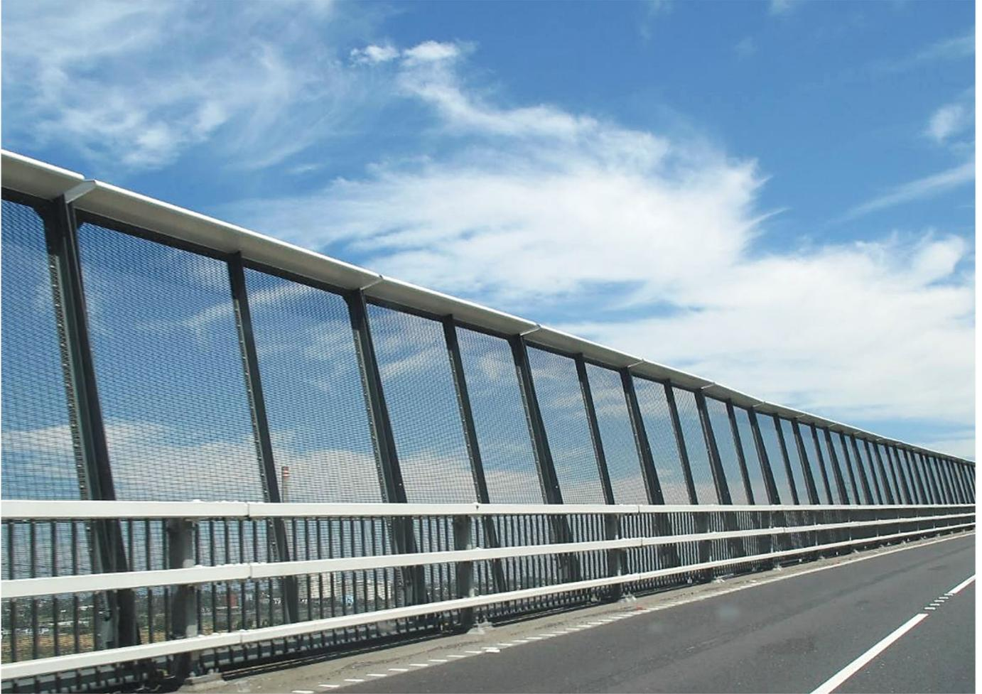
*Figure 1 – West Gate Bridge – Public Safety Barrier (Melbourne, Victoria)*
