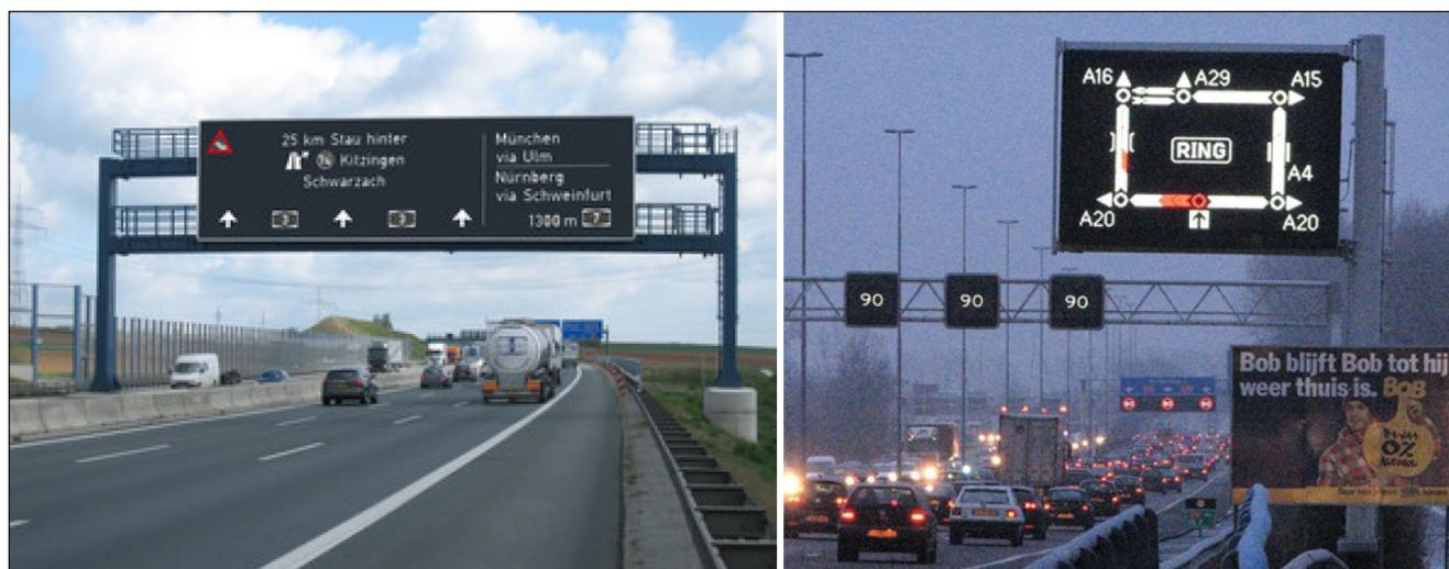
**Figure 4.1 A SWARCO full matrix LED sign in Bavaria, Germany (left) and a full matrix LED sign in Holland (right)**
