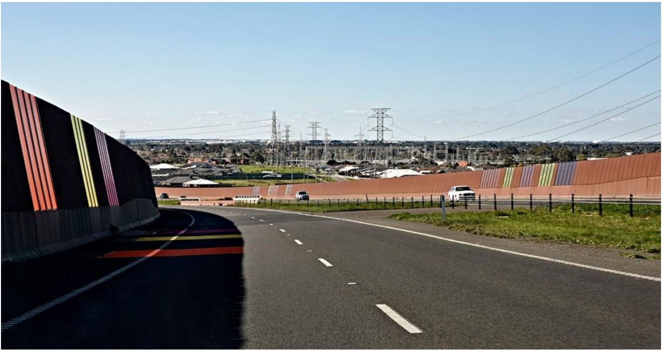
Figure 14 – Construction and materials, example of weathered steel and a painted approach to avoid visible staining of concrete road barriers, Geelong Ring Road (Geelong, Victoria) (Image source: Wood Marsh Architects)
