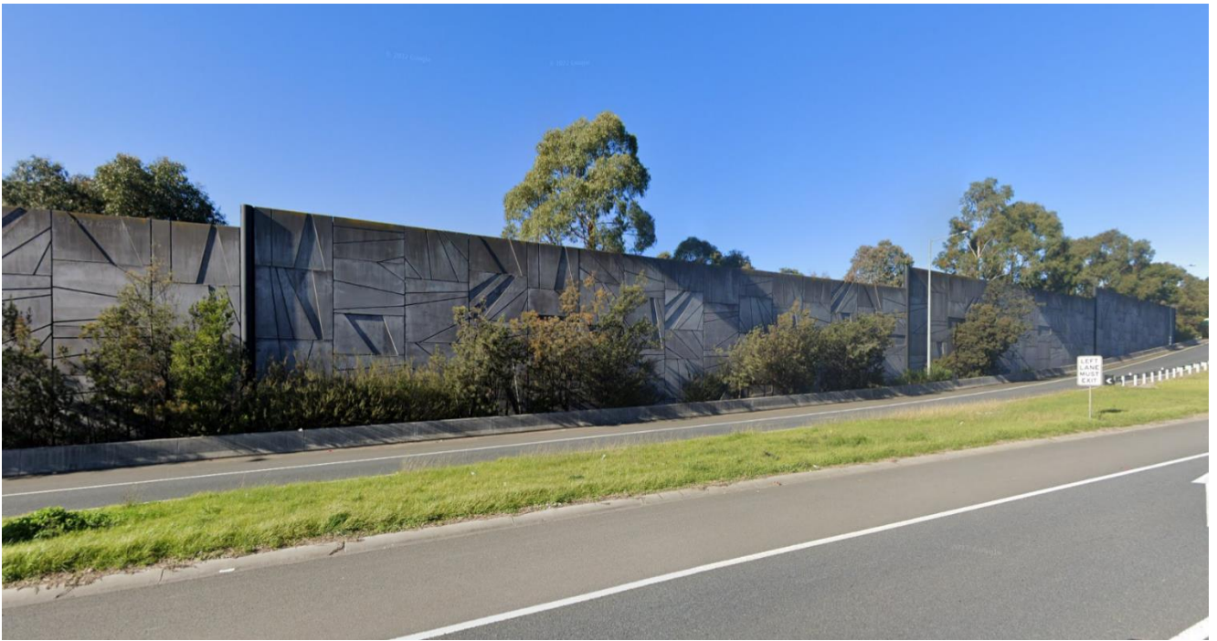
Figure 15 – Construction and materials, example of concrete noise wall with stepping, Eastlink (Dandenong North, Victoria) (Image source: Google Maps)
