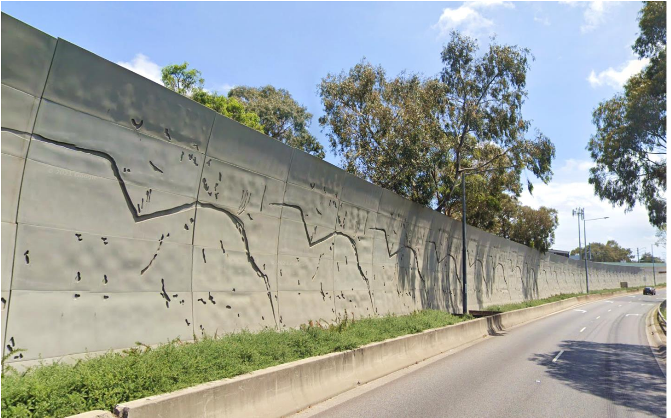
Figure 13 – Construction and materials, example of concealed noise wall posts and use of recycled materials, Monash Freeway, (Kooyong, Victoria) (Image source: Google Maps)
