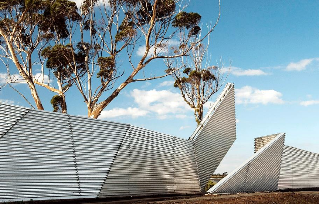
Figure 19 – Safety and Maintenance with well-considered noise wall overlaps providing access, Western Freeway (Deer Park, Victoria)
