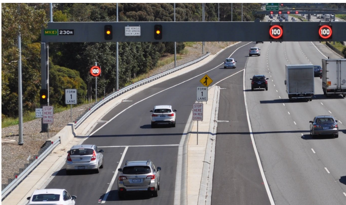
Figure 8-5: Freeway Ramp Signals – Including Ramp VSL Integration with Mainline LUMS and Co-location of ITS Assets
