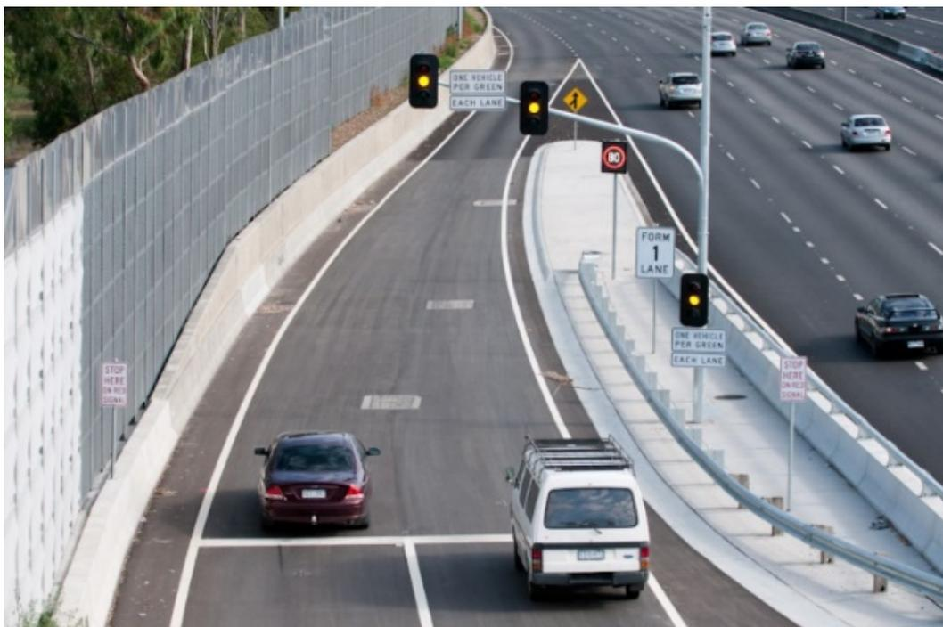
**Figure 2-1: Motorway Ramp Metering**
