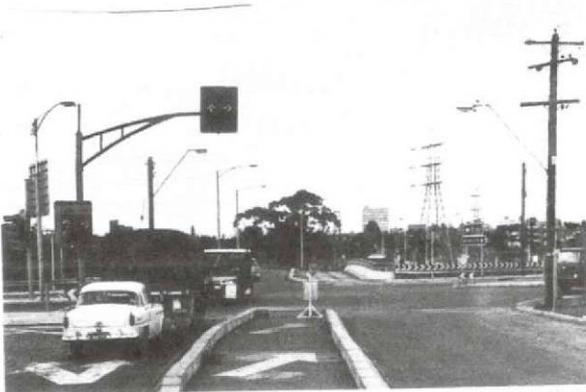
FIGURE 3. Traffic signal display at the intersection of the local streets and the Gibdon Street On Ramp to the South Eastern Freeway.
