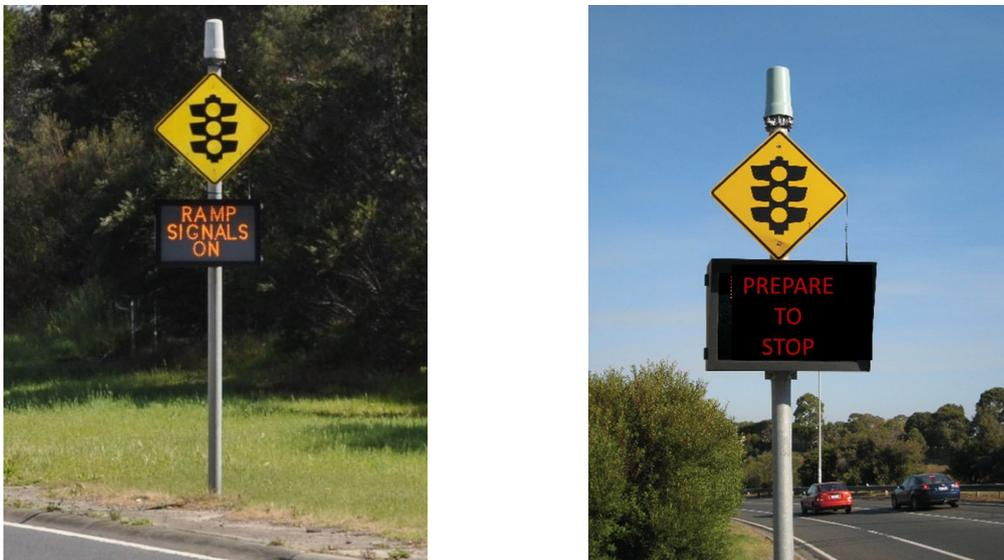
**Figure 6-13: RC2 Entry Ramp Warning Signs with Alternating Messages**
