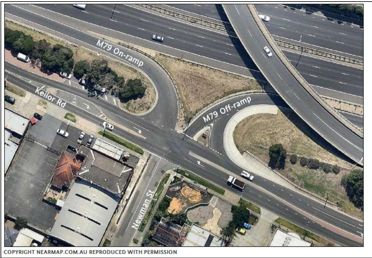
Figure 11: Aerial photo of Keilor Road/Newman Street (Source: Nearmap)
