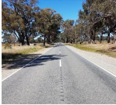
**Photo 4: ATCL Two-Way Barrier Line with black ribs**
