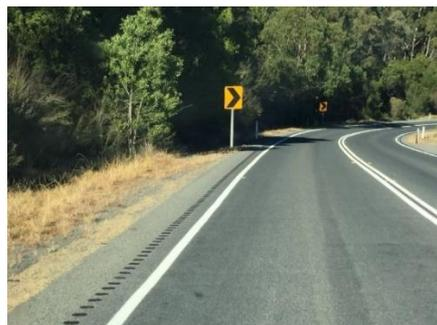
0.5m is the absolute minimum sealed shoulder required for the installation of offset audio tactile ribs. This allows for the minimum 0.3m recovery area behind the audio tactile ribs.
