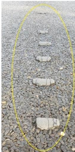
Issues may occur with shattering of audio tactile ribs due to installation during extreme temperature. Installations on hot days may not allow enough time for the adhesive to harden so that the audio tactile ribs may pluck when trafficked. The opposite occurs on cold days where the tactile hardens before it adheres to the surface. The construction team need to check with the manufacturer about the specifications for temperature at the time of installation.
