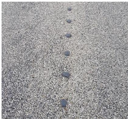
On some older seals, issues have been found with adhesion of audio tactile ribs to the existing seal.
