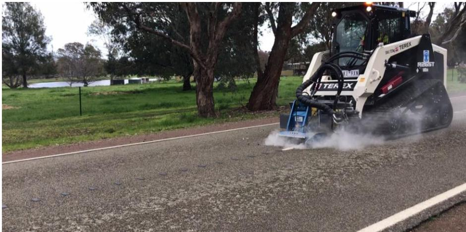
Grinding off audio tactile ribs is the preferred method of removal and has been proven to have a good result post removal. Other methods of audio tactile rib removal may be used but consideration must be given as to how this may impact or damage the pavement.
