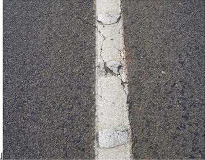
Cracking of the existing seal along the crown or edge line can cause premature failure and plucking of audio tactile ribs.
