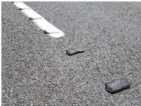
8mm high x 100mm long x 50mm wide white audio tactile ribs at 250mm centres should be used for WCLT.
