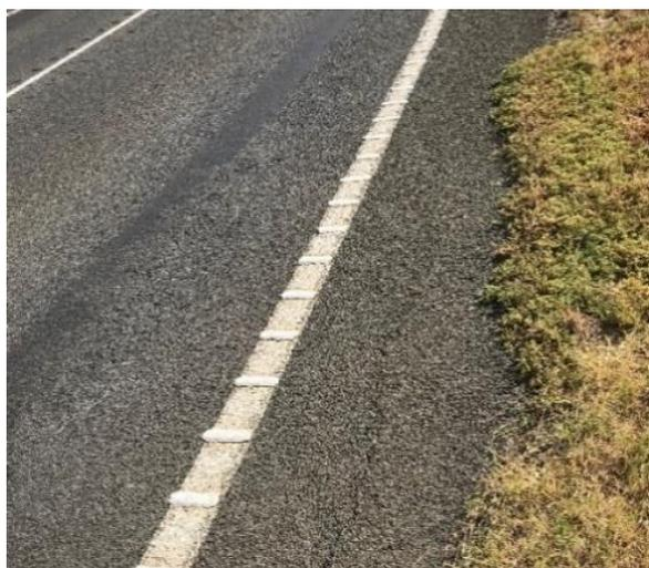
**Figure 4: Retrofit ATEL Installation - Absolute minimum sealed shoulder 0.35m with on-line audio tactile ribs**
