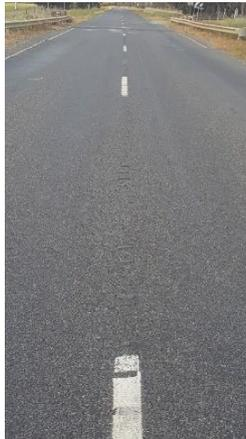
Issues with durability of audio tactile ribs have been found on some installations where the mixture for the audio tactile ribs has led to an unacceptable rate of premature failure (either by plucking or shattering of ribs).
