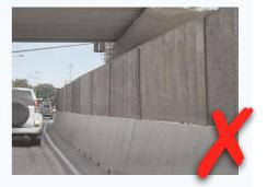
Timber panels erected on PCBs. The vertical cover strips between panels present a potential hazard to road users.
