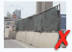
Temporary fence panels mounted on PCBs. Horizontal rails constitute a potential spearing hazard and are not permitted.
