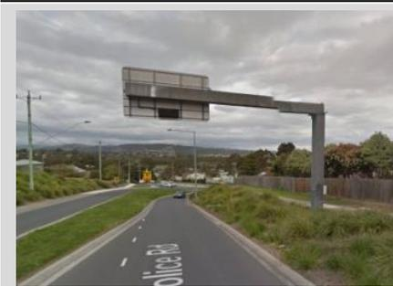
This cantilever support has a low probability of collapse given the elevated location and 60km/h likely impact speed. In this case, there is a very low chance for collapse or fatal and serious injuries.
