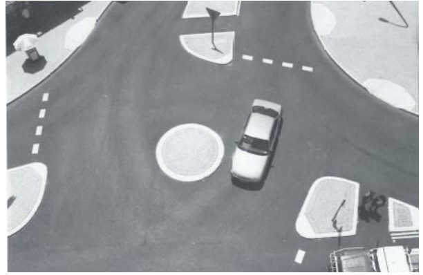
Aerial View – note the small fully mountable central Island.
