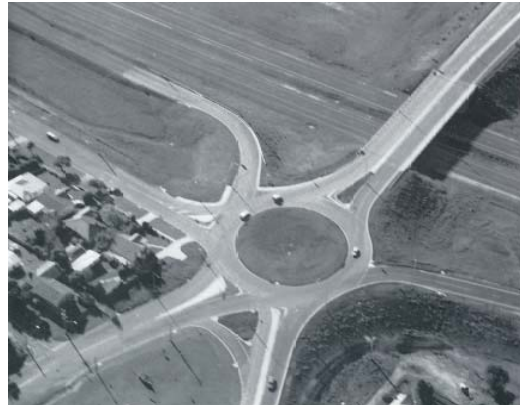
Freeway Interchange Roundabout Warragul Victoria
