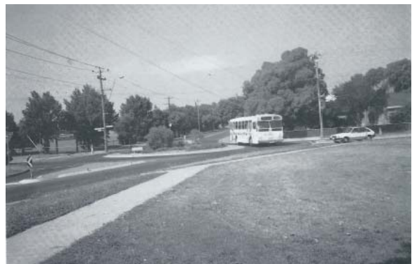
Note Bus encroachment on to central island.
