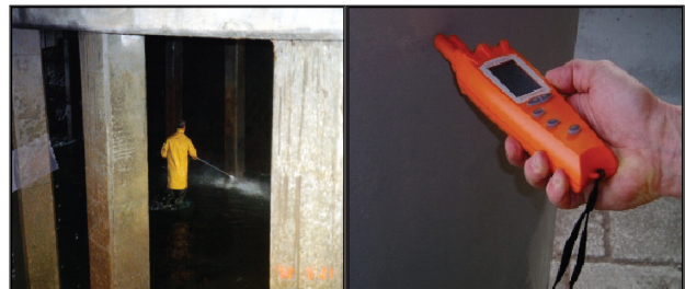
Fig. 2 Preparation of the concrete surface for coating application (L), Measurement of relative humidity, dew point and temperatures (R)
