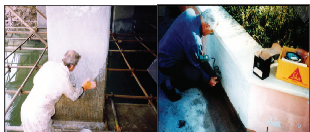
Fig. 4 Application of epoxy coating by hand (L), Moisture meter in use (R)
