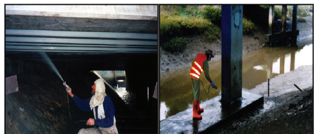
Fig. 3 Spray application of anticarbonation coating (L), Application of silane with fugitive dye on 3 year old bridge as part of preventative maintenance (R)
