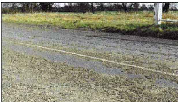
Figure 1: Loss of Aggregate
