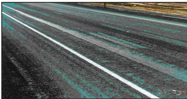
Figure 2: Stripping in new work
