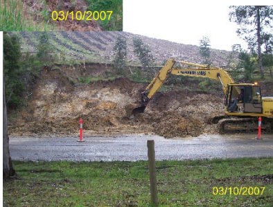
Figure A2: Landslide (rotational failure).
