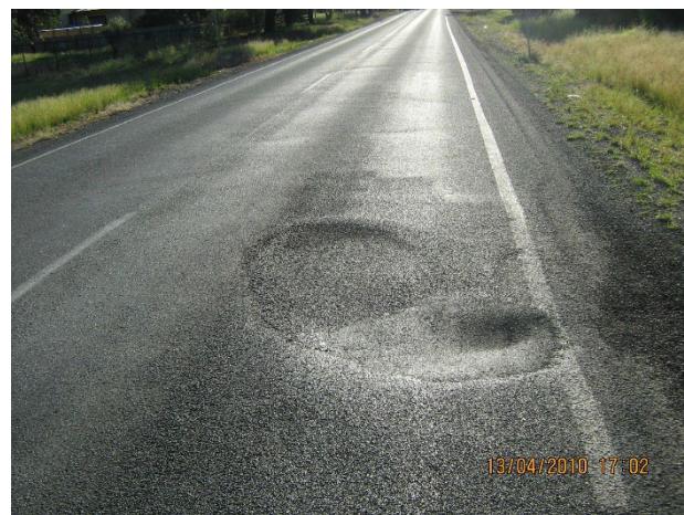
Figure A10: Subsidence (pavement settlement).
