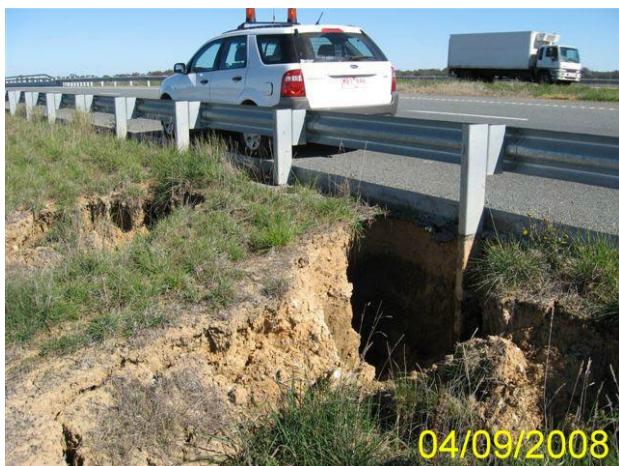
Figure A7: Erosion (cavity created by piping).
