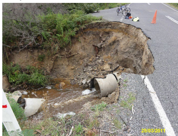
Figure A6: Erosion (erosion at culvert outlet).
