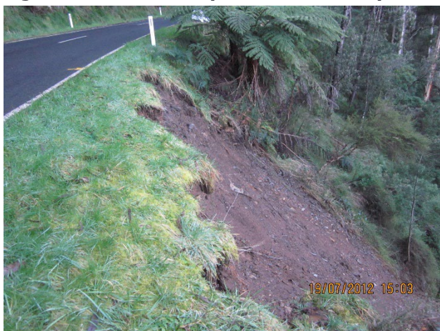
Figure A3: Landslide (slumping of soil).
