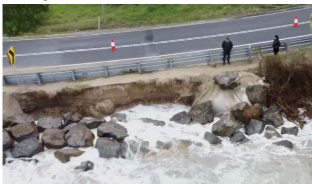
Figure A9: Coastal processes (erosion by wave action).
