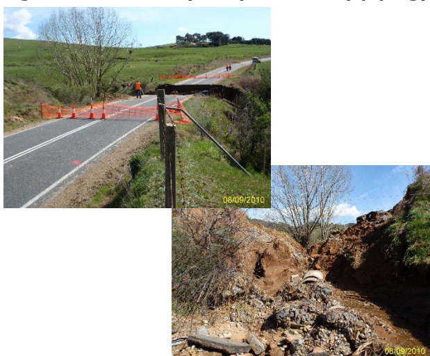
Figure A8: Erosion (embankment fill acting as a dam).
