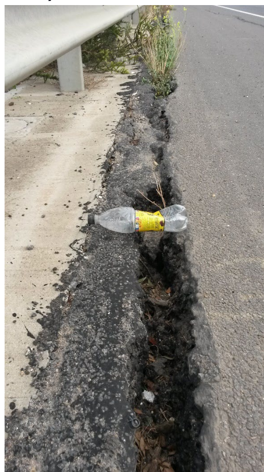
Figure A11: Expansive soil processes (cracking extending through the pavement, capping layer and subgrade).
