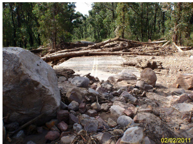
Figure A4: Landslide (debris flow).
