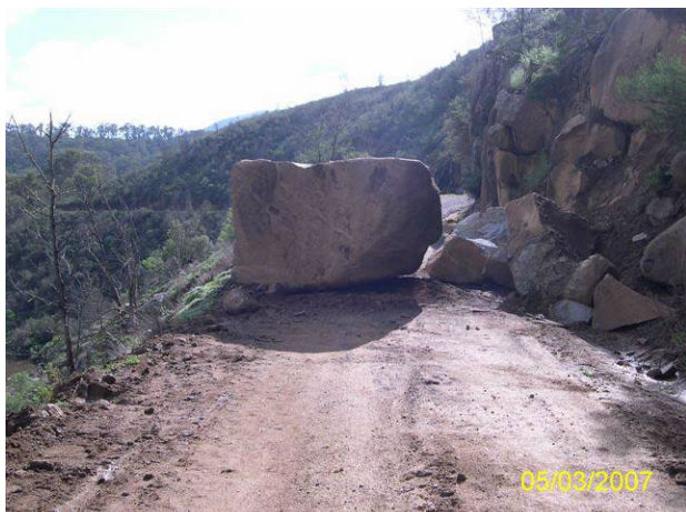
Figure A1: Landslide (rockfall).
