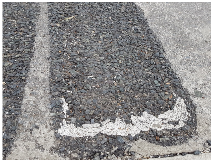
Figure 2: Asphalt surface damaged by marking removal
