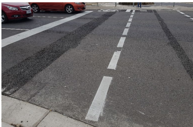
Figure 1: Ghost marking due to highly textured surface following marking removal
