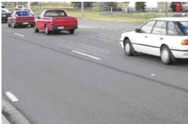
Figure 3: Marking removed by High Pressure Water Retexturing
