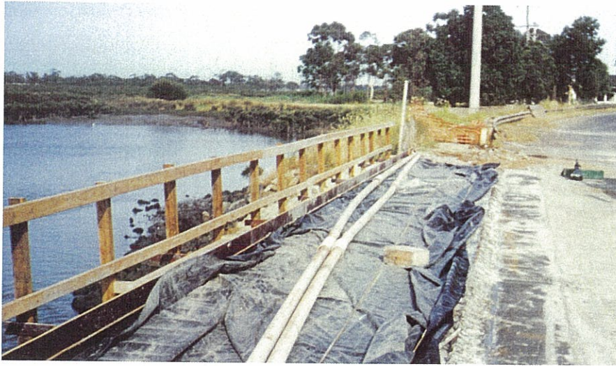
Fig. 3.5 Curing with Polyethylene Sheetting
