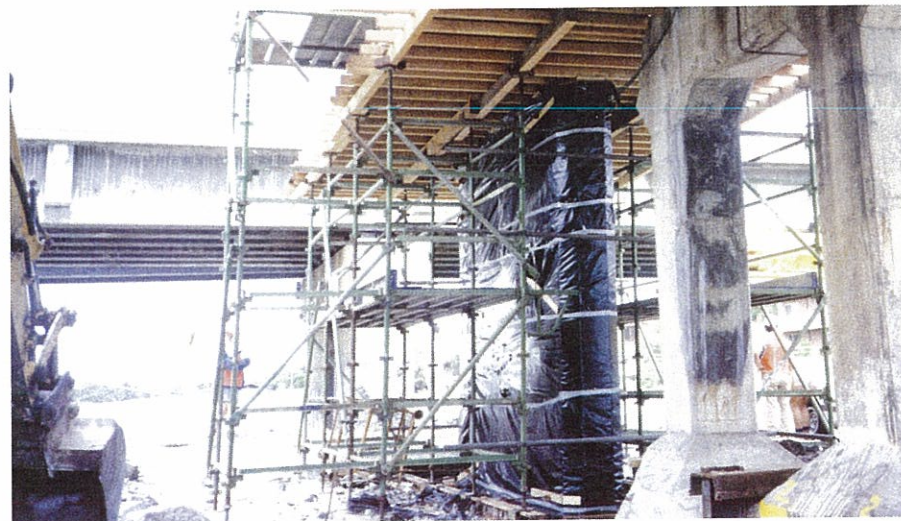
Fig. 3.8 Polyethylene sheeting effectively wrapped around component in marine environment
