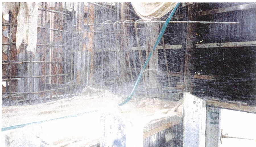
Fig. 3.1 Moist Curing of In-Situ Concrete via Sprinkling of Water
