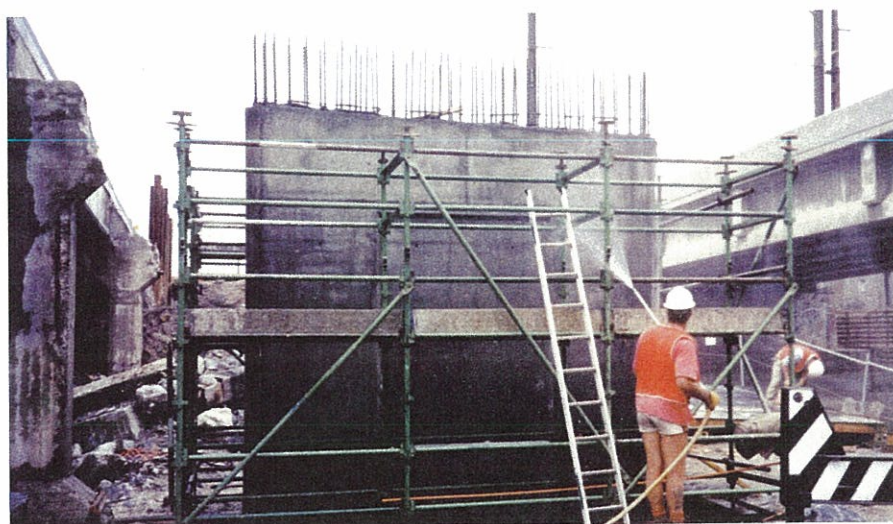
Fig. 3.4 Application of water spraying upon removal of formwork while awaiting the application of other curing
