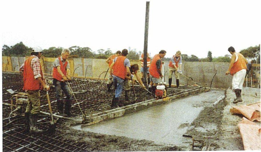
Fig. 3.7 Placement/Finishing of concrete with polyethylene plastic fixed on frame awaiting placement
