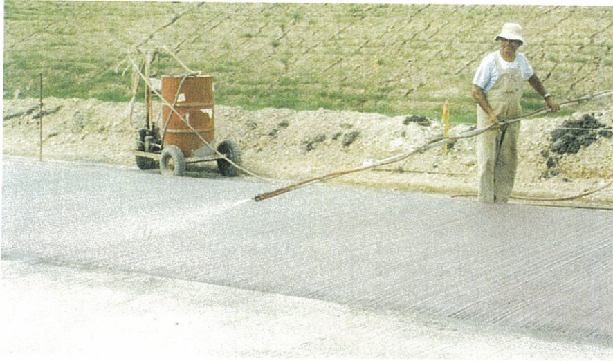
Fig. 3.9 Curing Compound Spray applied on finished concrete surface
