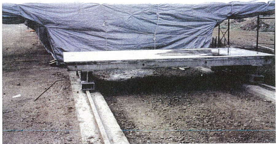
Fig. 3.12 Precast Component Effectively Sealed subsequent to Partial Steam Curing
