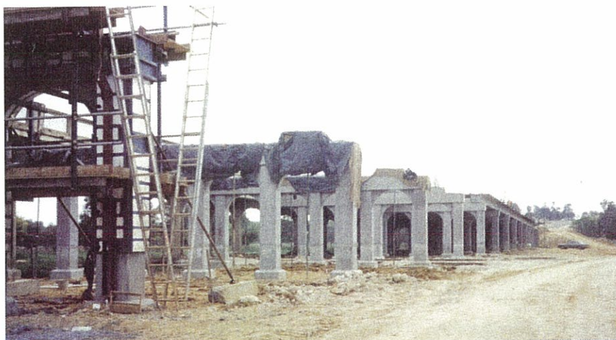
Fig. 3.3 Curing Blanket utilising Wet Hessian and Polyethylene Plastic over the top
