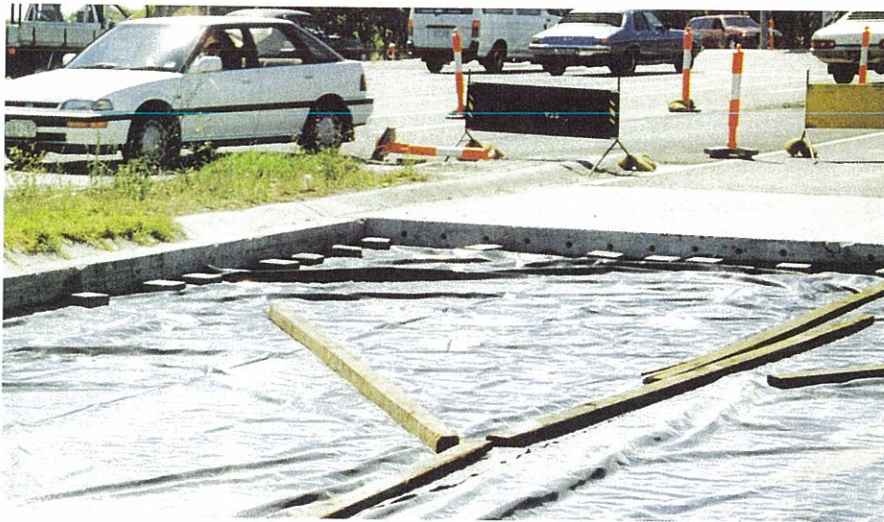
Fig. 3.6 Polyethylene Sheetting secured appropriately
