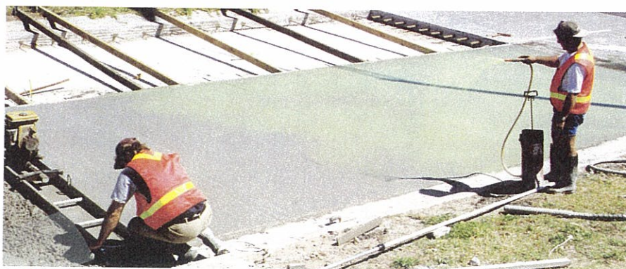
Fig. 5.1 Application of aliphatic alcohol (evaporative retarder) immediately after initial screeding
