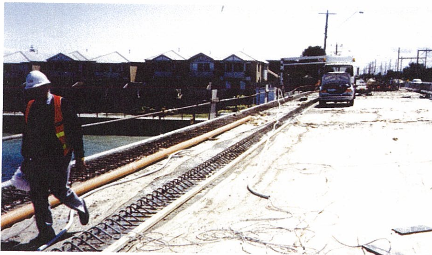
Fig. 3.2 Moist Curing with Wet Hessian
