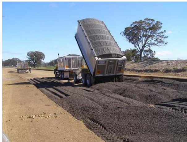
Figure 2 : Delivery of Material with Covered Trucks
