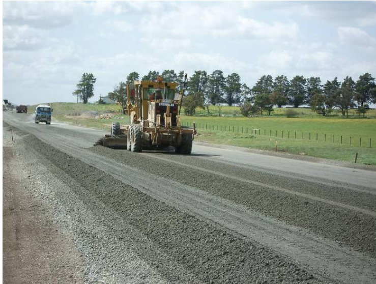
Figure 3 : Uniform Spreading of Wetmix Material
