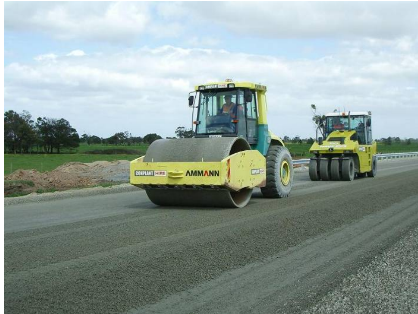
Figure 5 : Roller Routine using Steel and Pneumatic Tyred Rollers
