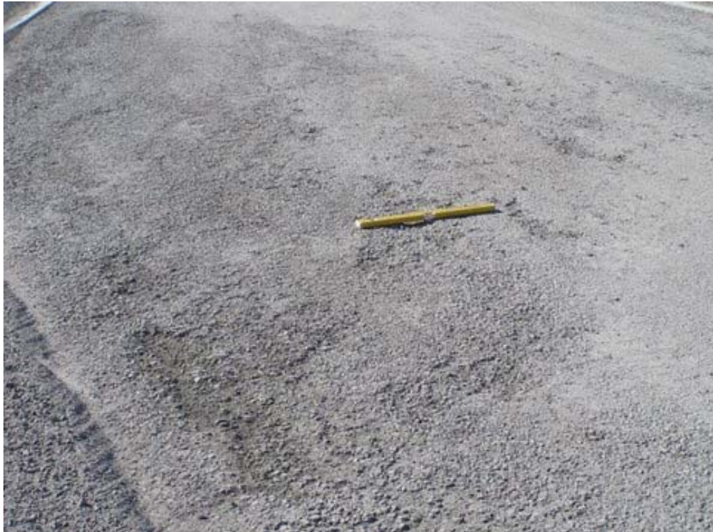
Figure 8 : Ravelled Area following Brooming
