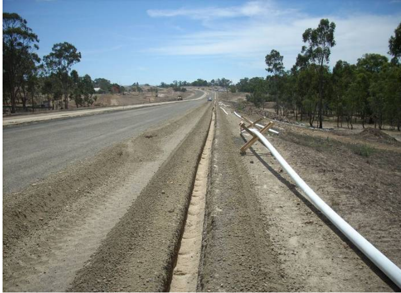
Figure 6 : Low Side Subsurface Drain
