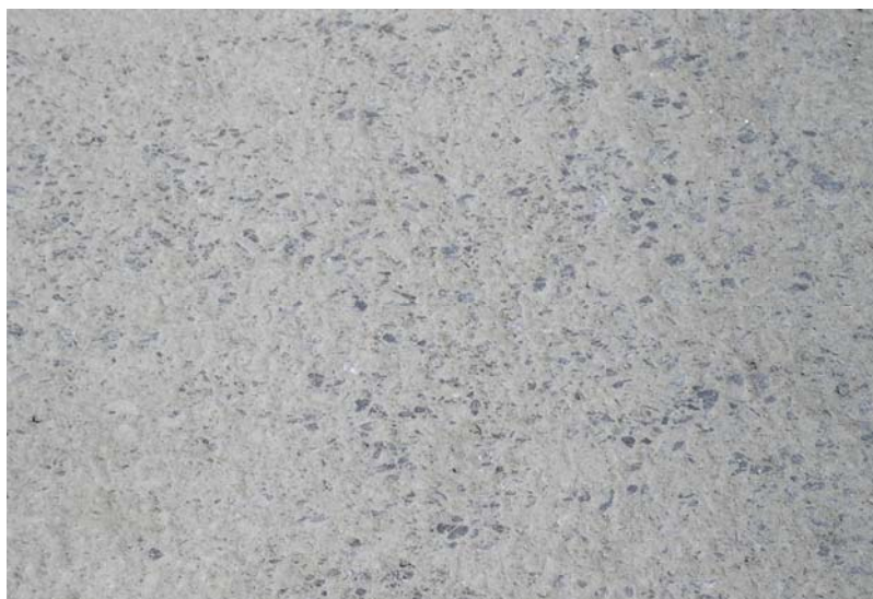
Figure 7 : Well Prepared Surface
