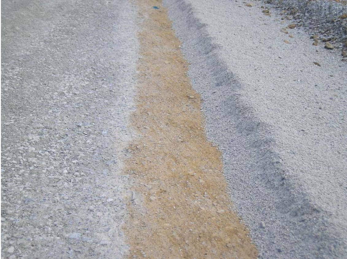
Figure 1 : Surface Lacking Cohesion during Brooming
