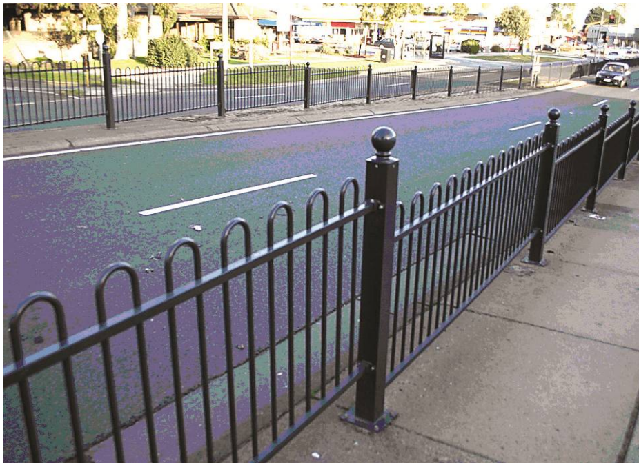
Example of pedestrian fencing
