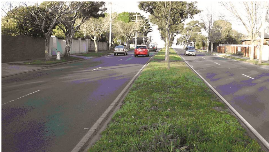
Example of a Kerbed Median
