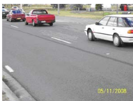
Figure 35: Removal of pavement markings using High Pressure Water Blasting
