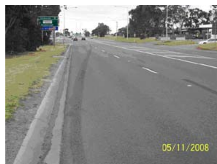
Figure 35: Removal of pavement markings using High Pressure Water Blasting
