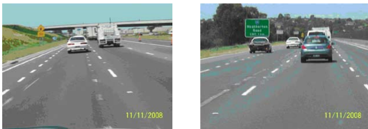
Figure 36: Examples of ineffective removal of redundant lines using grinding process.
