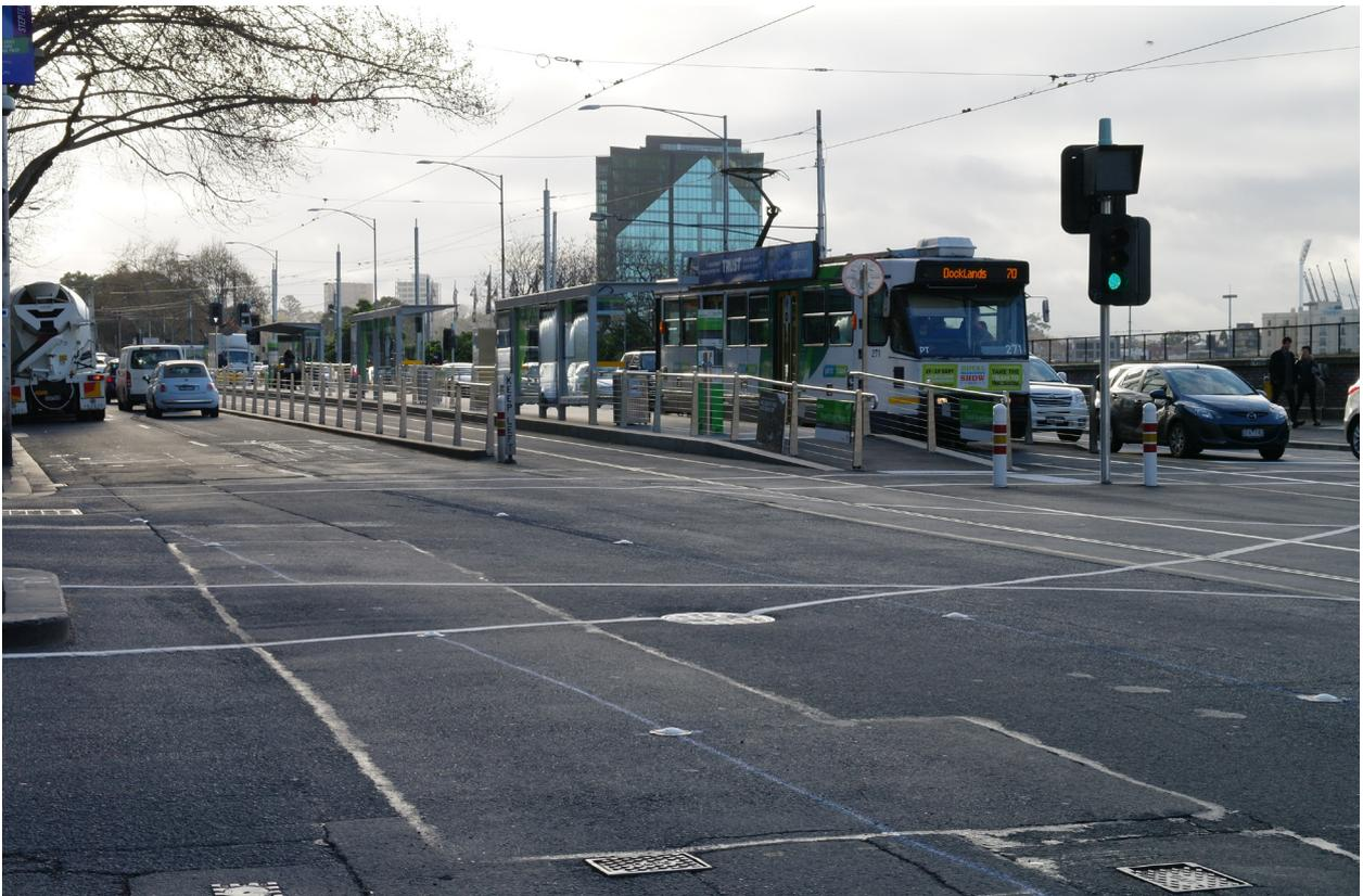
**Figure 24: Centre island platform stop, no vehicular traffic adjacent to tram tracks – Flinders St / Russell St, Melbourne**
