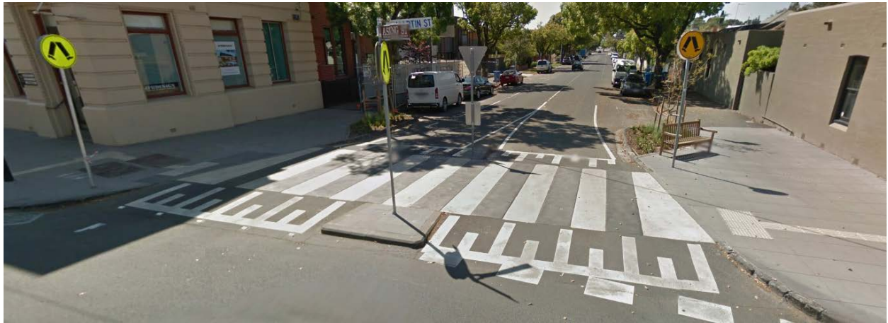
Figure 42: Raised pedestrian crossing at the roundabout holding line - Asling Street and Martin Street, Brighton. Note the pedestrian crossing signs have been angled to face circulate traffic. Image source: Google Maps
