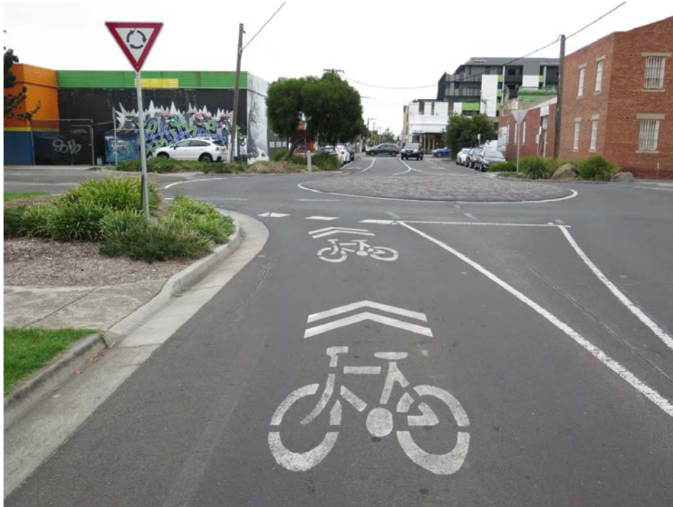
Figure 24: Example of sharrow pavement markings at a roundabout on Highett Street, Richmond
