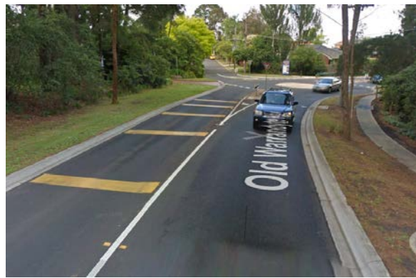
Figure 30: Flush transverse lines
