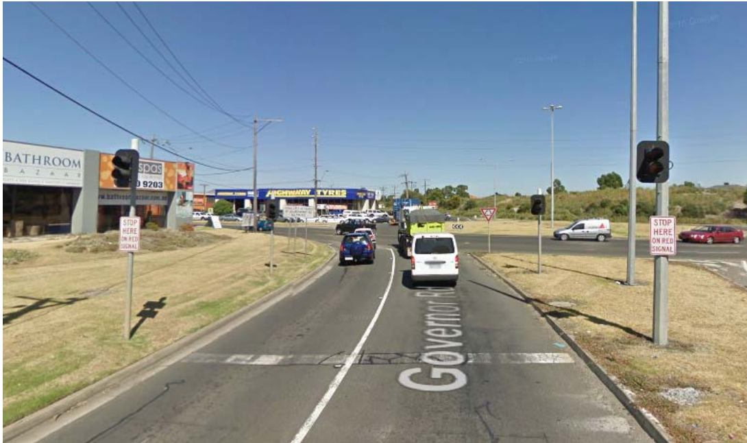
Figure 35: Metered roundabout approach at Governor Road and Boundary Road, Mordialloc. Image source: Google Maps
