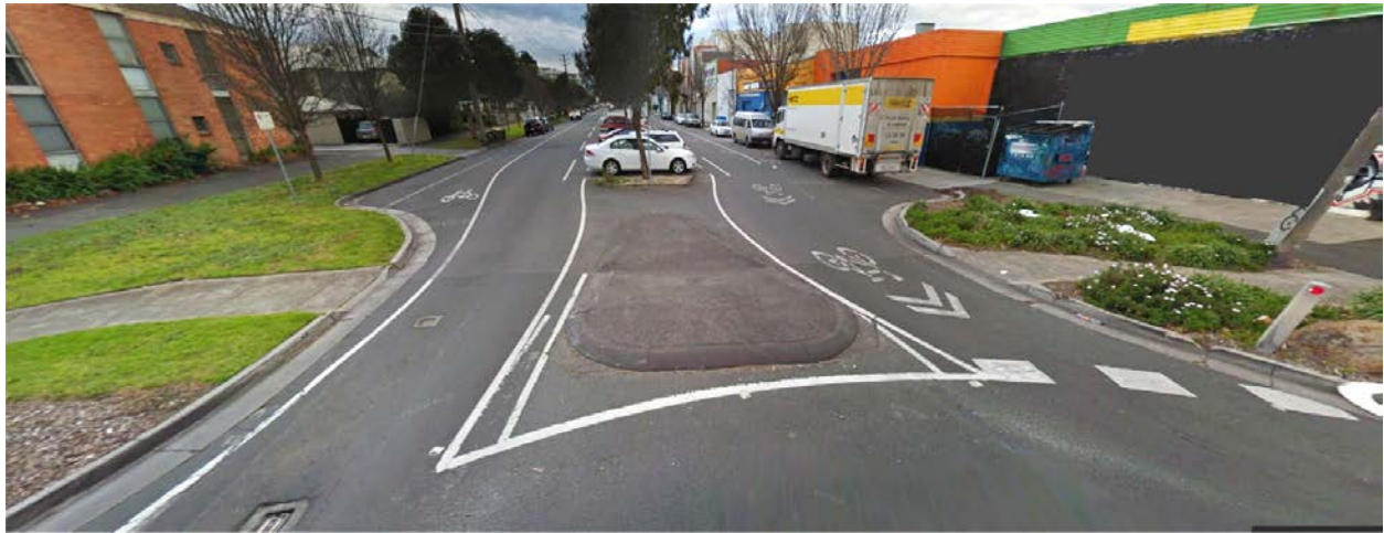
Figure 40: Kerb extensions at a roundabout in Richmond (note: DDA components are not shown in the image). Image source: Google Maps
