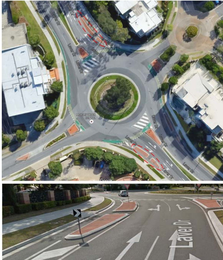
Figure 17: Splitter kerbs at Laver Drive and Easthill Drive roundabout in Robina, Queensland. Image Source: Google Maps
