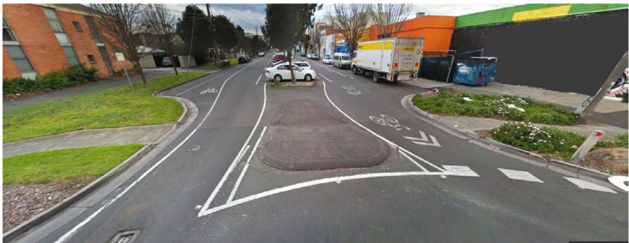
Figure 39: Local road roundabout with pedestrian refuge (note: DDA components are not shown in the image). Image source: Google Maps
