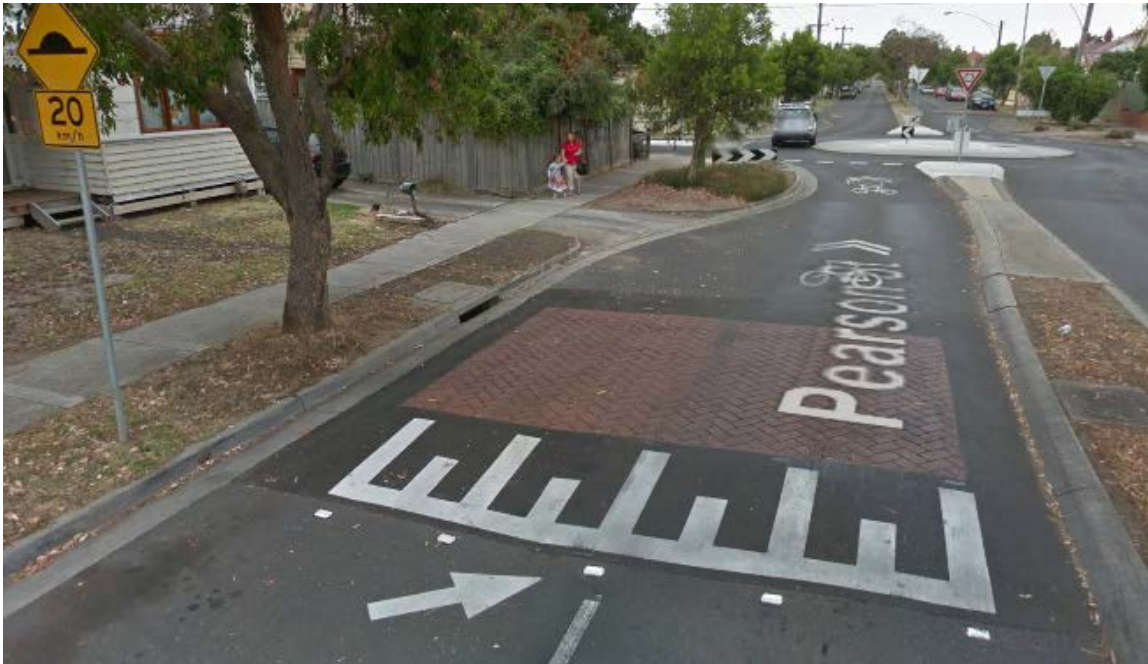
Figure 21: Flat top speed hump followed by sharrows on Pearson Street, Brunswick West. Image Source: Google Maps
