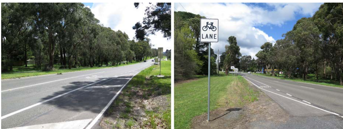
Figure 26: Approach to roundabout on Mountain Highway
