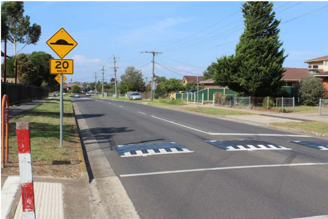
Figure 20: Example of a speed cushion
