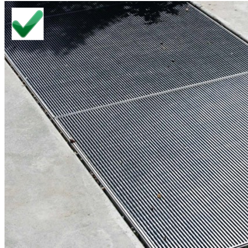
Figure 19: Grate with suitably sized openings
