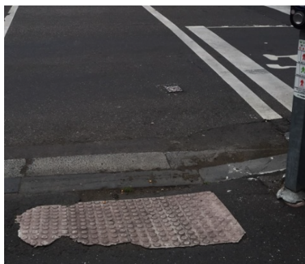
Figure 39: TGSIs luminance contrast and integrity not maintained
