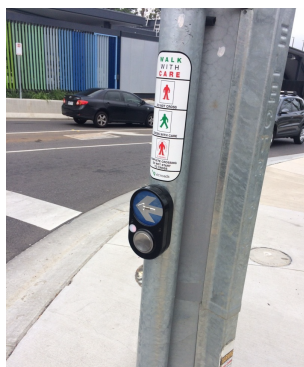
Figure 40: Push button assembly
