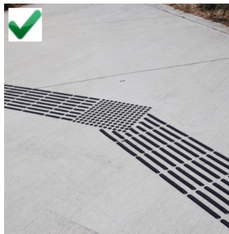
Figure 38: Tactile studs with sufficient luminance contrast to their base surface
