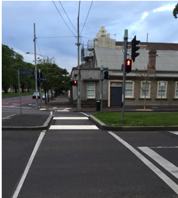
Figure 27: Median with cut through (in lieu of kerb ramps)
