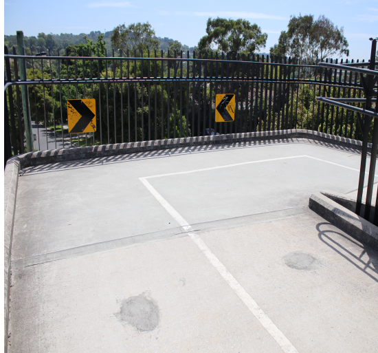
Figure 11: Turning space at a pedestrian overpass
