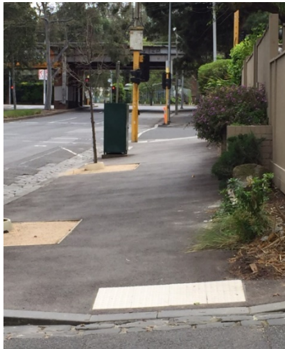
Figure 15: Footpath with crossfall exceeding 1:40 / 1:33
