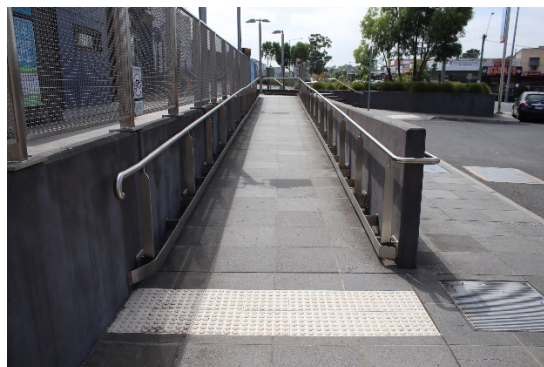
Figure 20: Ramp with compliant handrails
