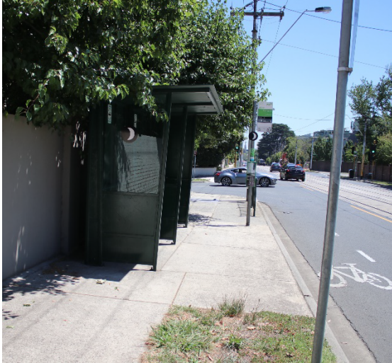
Figure 10: Turning space around a bus shelter
