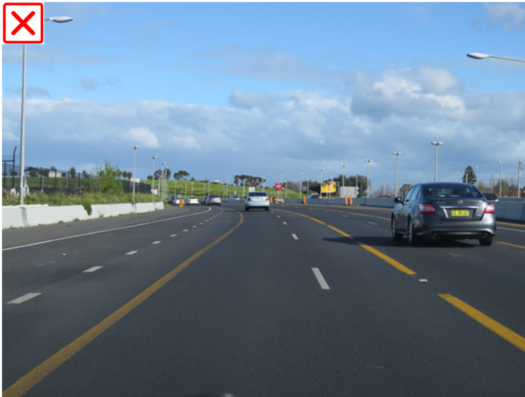
Figure 9: Example of faded temporary yellow linemarking - risk of confusion to motorists increases
