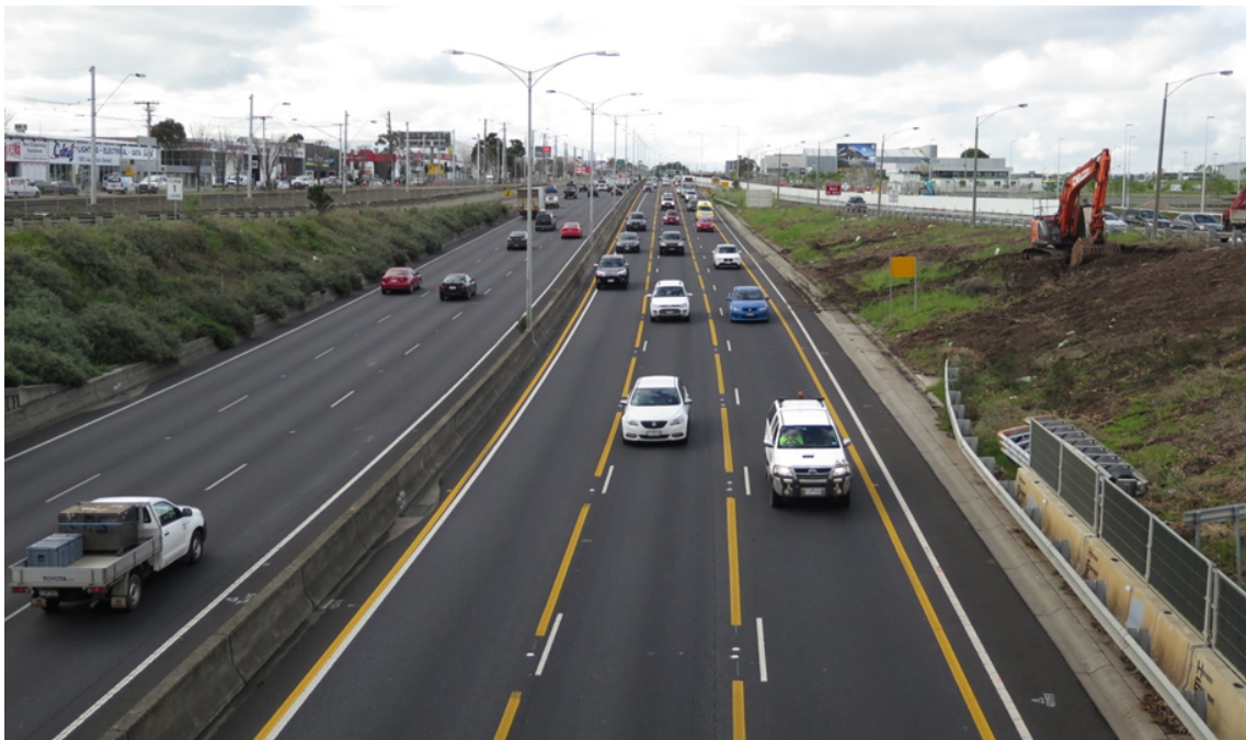
Figure 1: Temporary yellow linemarking (9 m yellow line with 3 m gap standard) on a freeway
