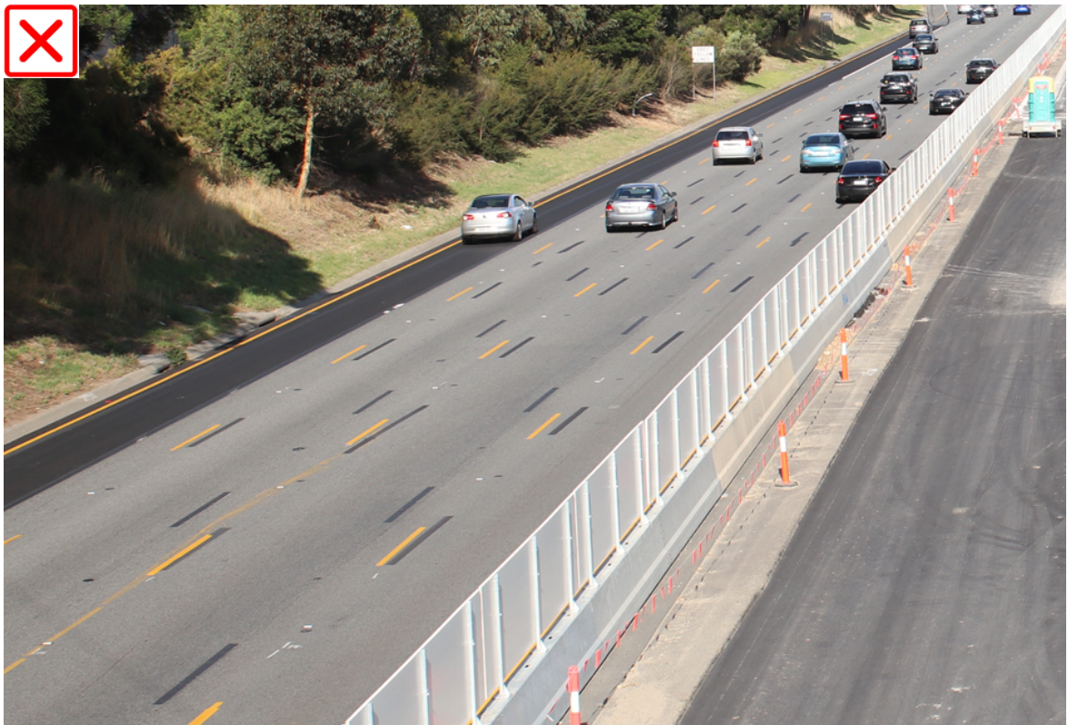
Figure 4: Example of "ghosting" effect as a result of a black covering material used on a light coloured pavement with a (substandard) 3 m yellow line, 100mm wide and 9 m gap treatment.
