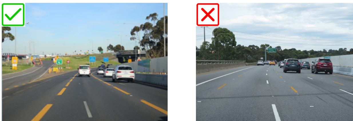
Figure 2: Comparison of 9 m yellow line, 3 m gap, 150 mm width (left; standard) to 3 m yellow line, 9 m gap, 100 mm width (right; substandard)
