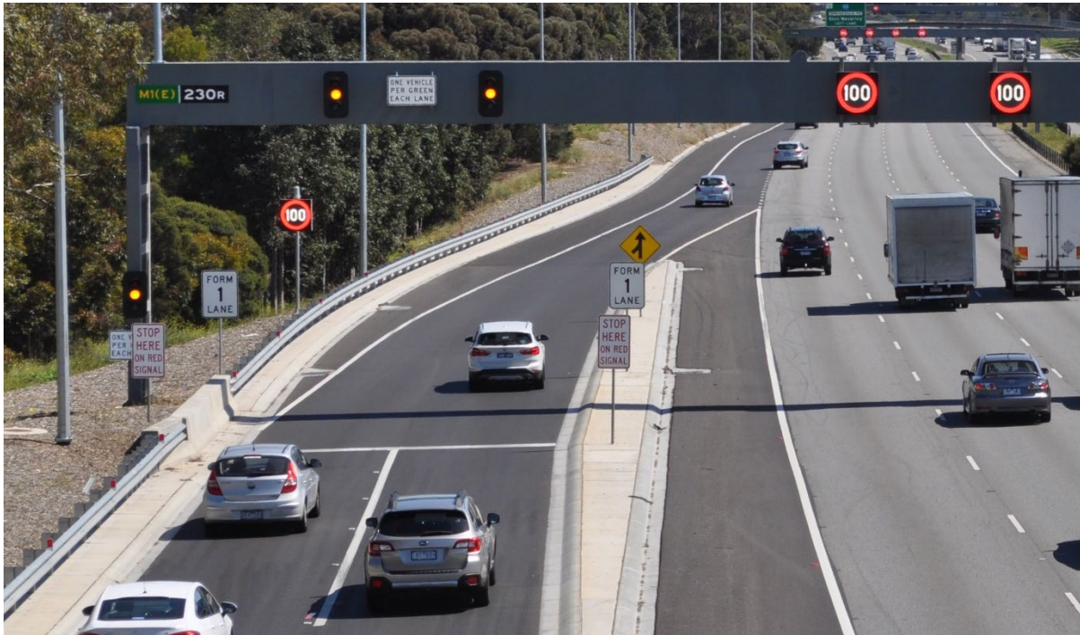
Figure 8-5: Freeway Ramp Signals – Including Ramp VSL Integration with Mainline LUMS and Co-location of ITS Assets
